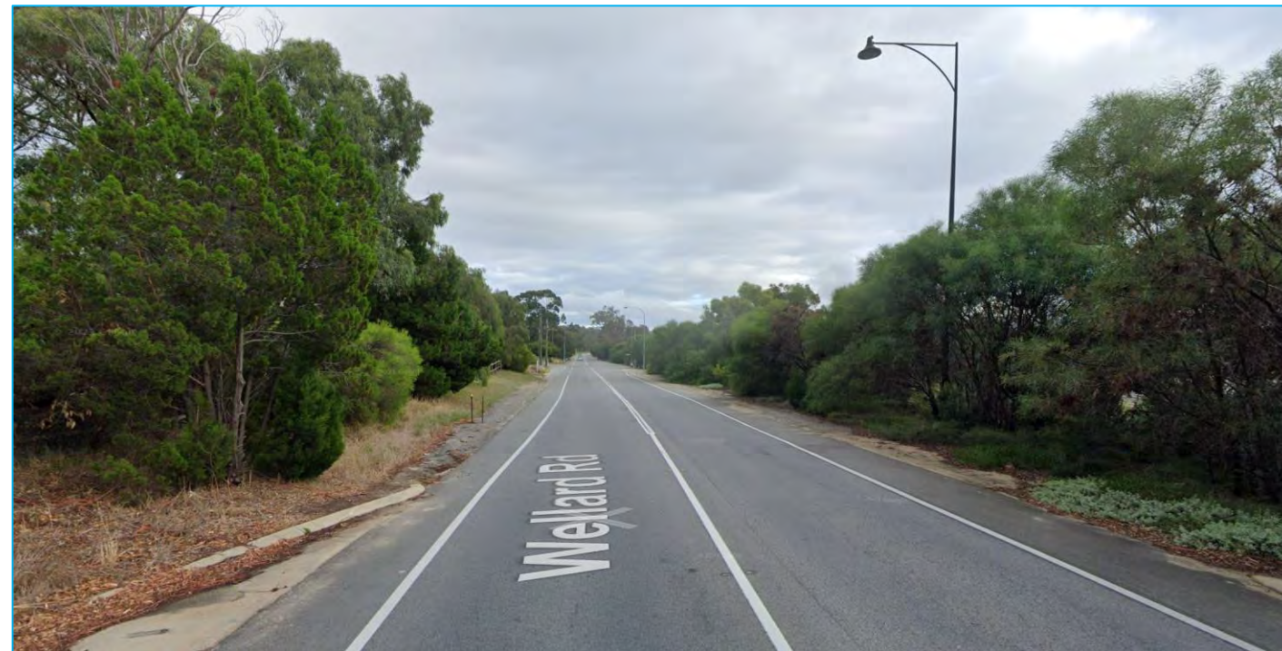
Figure 2-6: Typical Layout of Wellard Road – Looking north (north of Cavendish Boulevard)
