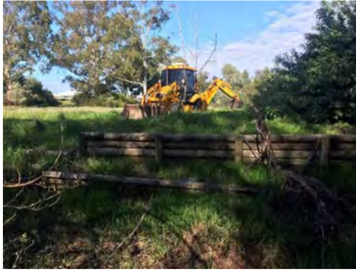
Plate 1: Small wooden retaining wall and associated elevated ground area adjacent to TP6
