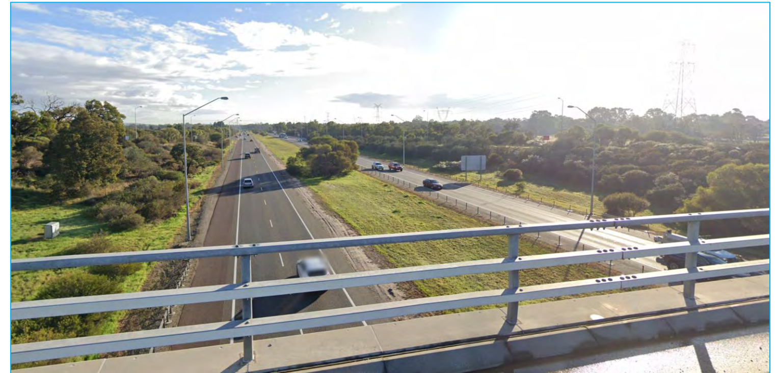
Figure 2-9: Kwinana Freeway – Looking north (north of Mortimer Road)
