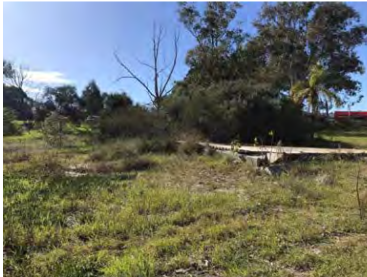
Plate 2: Old foundation slab
