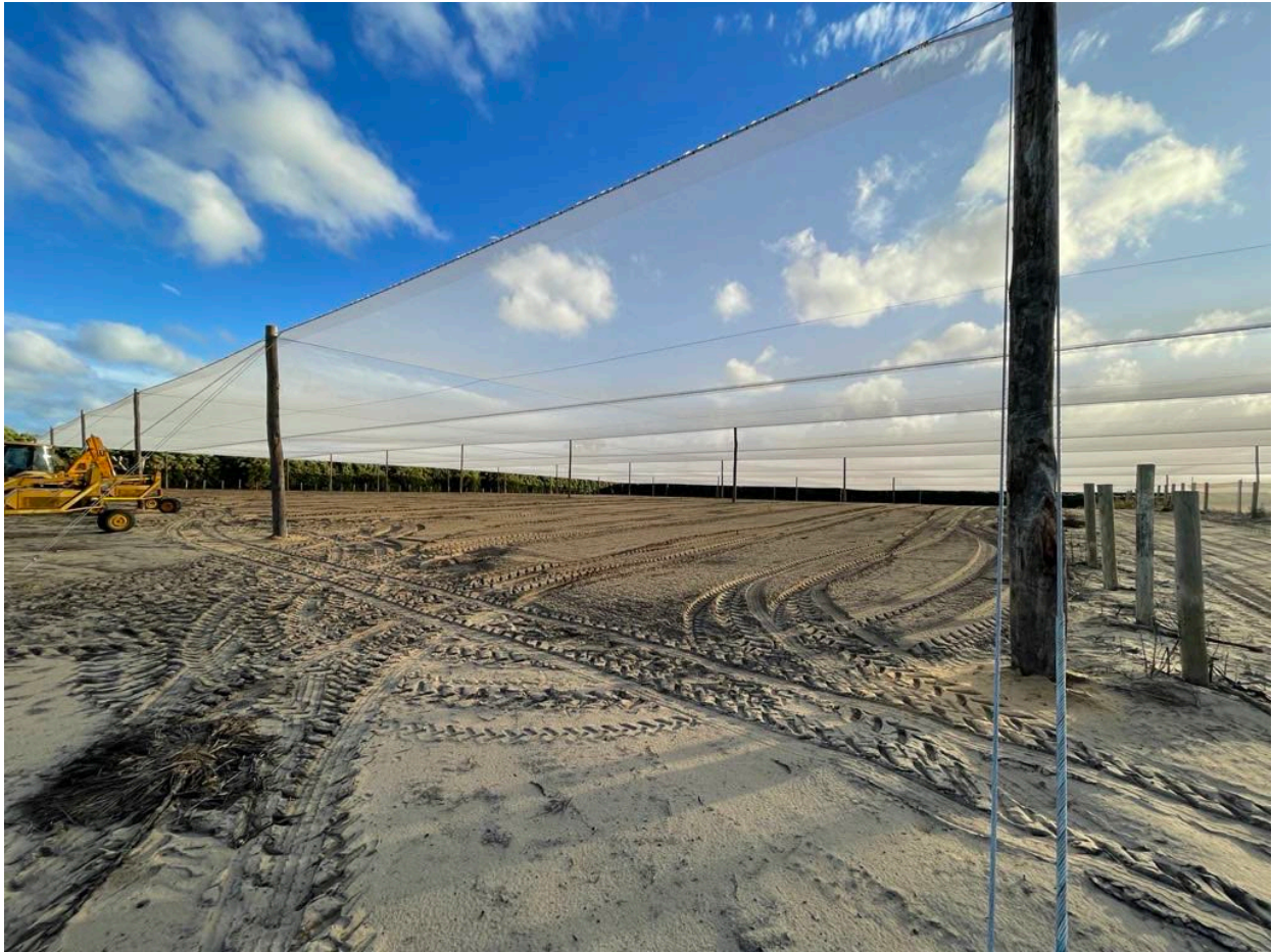
Figure 8 A net house installed using a grant under the Gngangara Water Use Efficiency Grants and Voucher Program to protect against crop loss, reduce evaporation and increase water use efficiency (Photo credit: DPIRD)
