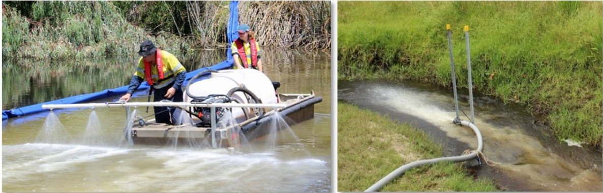
Figure 9-4 Clay application to stationary water (left) and to a flowing drain (right)
