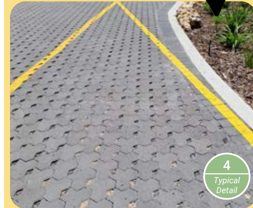
Figure 18. Permeable paving used in parking area provides additional deep soil for adjacent trees and planting. Source: Author.
