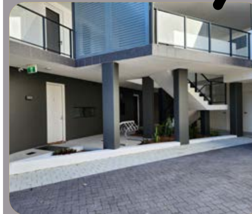
Figure 84. Communal open space is not integrated into project with over 10 units.
