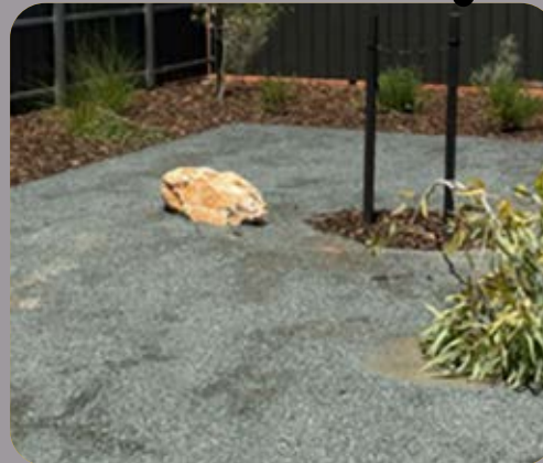
Figure 113. Cracker dust and rocks become too hot to sit on or use. Insufficient deep soil area for tree.
