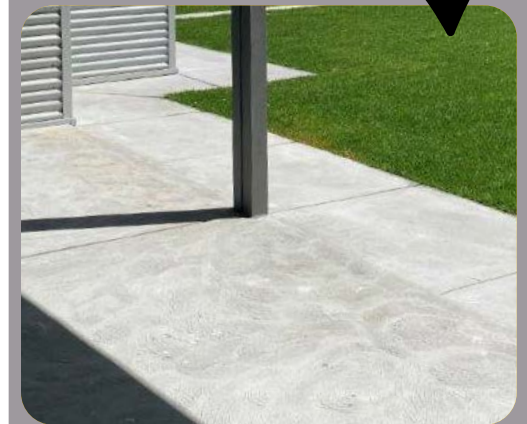
Figure 65. Light colour finish and lush transitions between alfresco, access paths and turf and passively drained.
