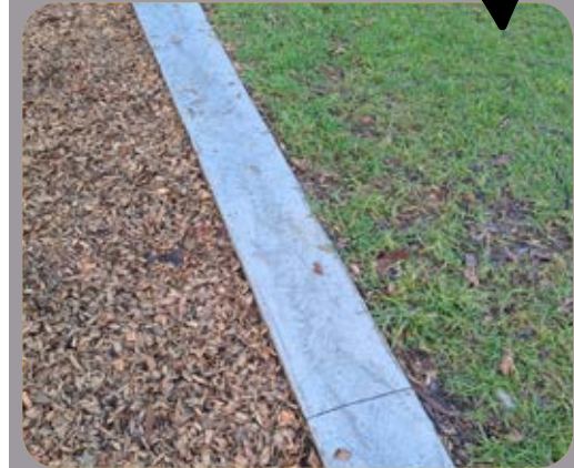
Figure 23. Flush and wide concrete edge provides a quality and robust edging.
