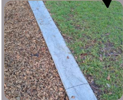
Figure 67. Flush and wide concrete edge provides a quality and robust edging
