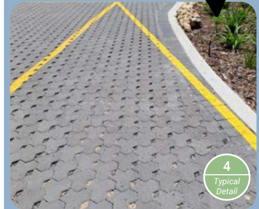
Figure 60. Permeable paving used in parking area provides additional deep soil for adjacent trees and planting. Source: Author.
