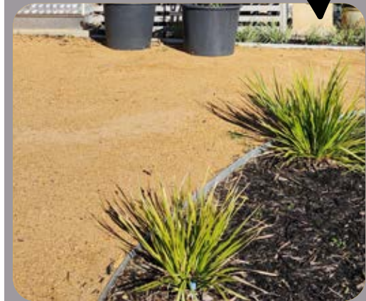
Figure 27. Gravel area is flat, contained with edging, balanced spatially with planting and has no weed penetration.
