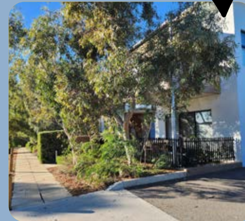
Figure 56. Trees planted in the front garden improve visual amenity and provide summer shading.
