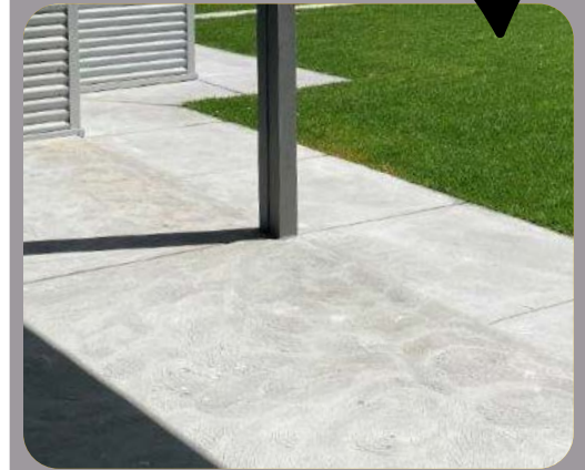
Figure 21. Light colour finish and flush transitions between alfresco, access paths and turf and passively drained.
