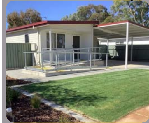
Figure 118. A balance of hard surfaces, turf and garden beds provided. Concrete edges separate turf and garden beds.
