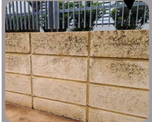
Figure 35. Limestone block with integrated boundary fencing is a preferred construction method.
