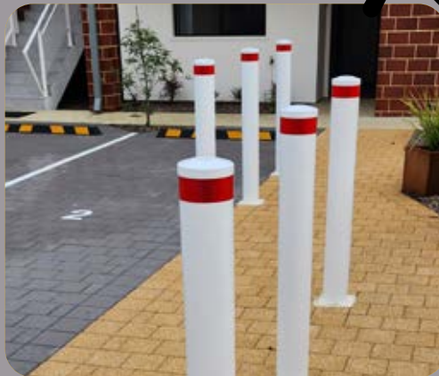
Figure 78. Vehicular bollards are to be avoided in favour of better site planning and design.
