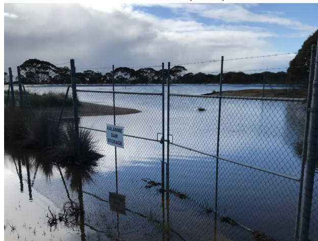
Kalannie Dam full (September 2022)
