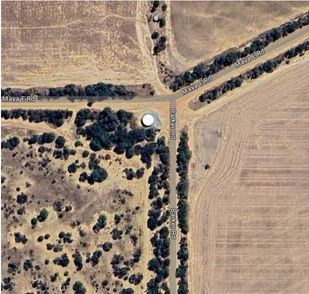
Maya East Road tank aerial
