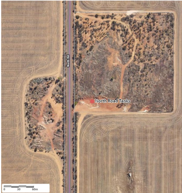
Aerial view of North Road tanks
