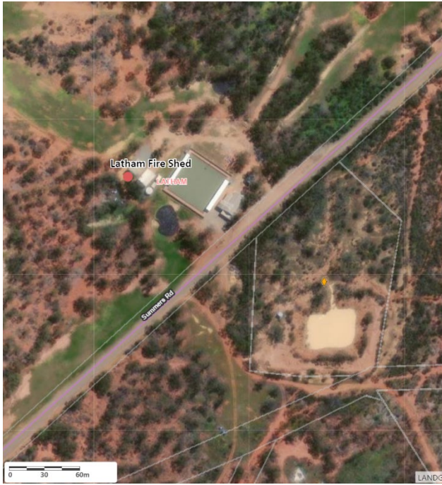
Fire shed tank aerial
