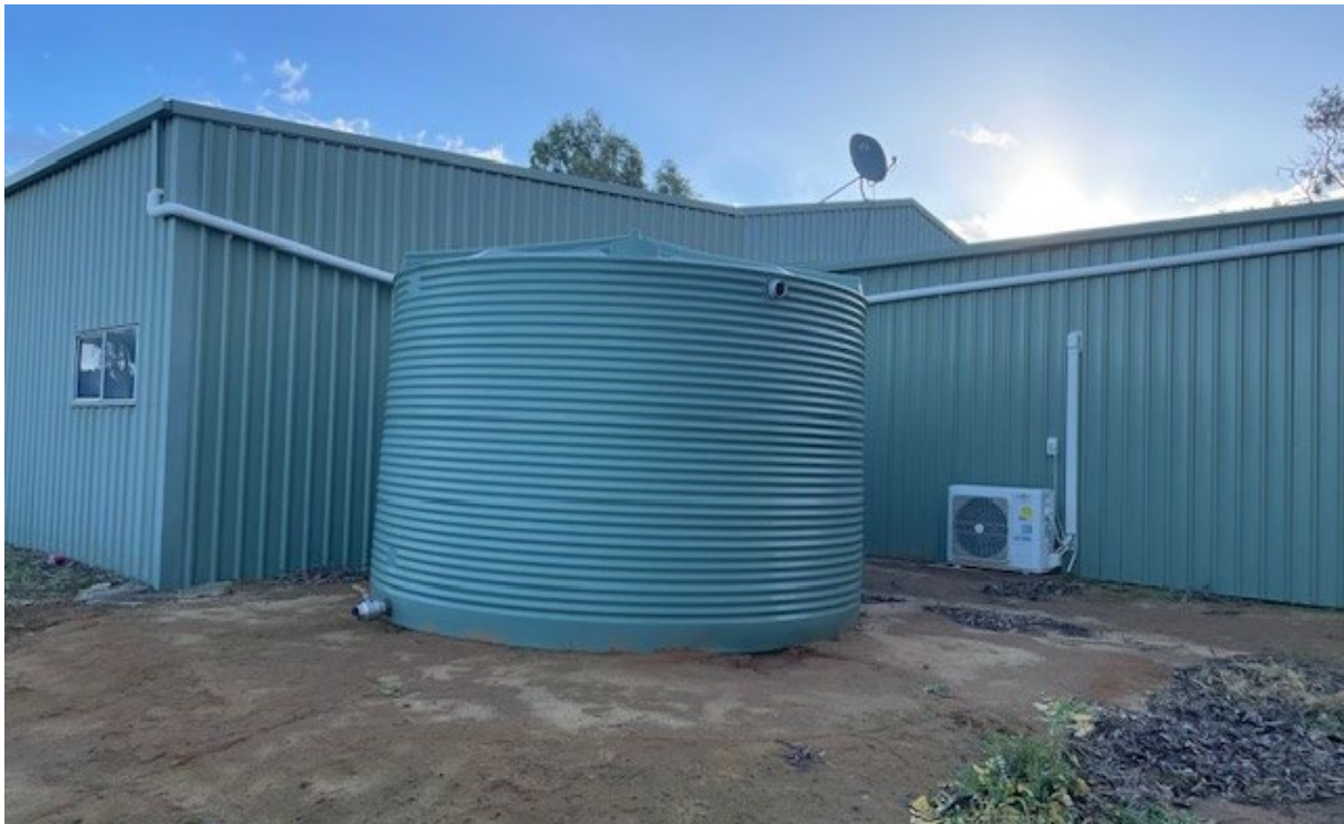
Fire shed tank
