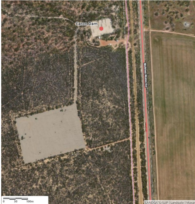
Aerial view of Caron Dam
