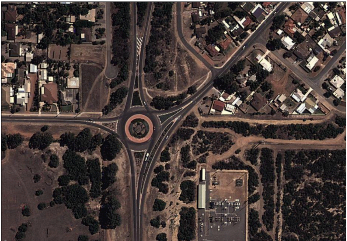
Figure 4 North West Coastal Highway / Chapman Valley Road Intersection
