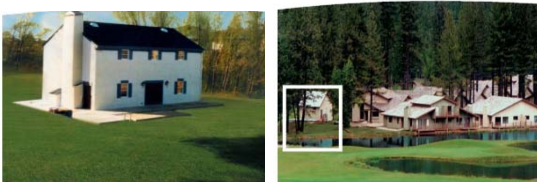
Plates 1 & 2: Example Aqueonics WWT facilities, West Chester PA, & Truckee, CA
