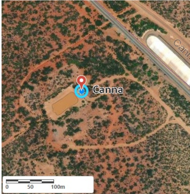
Aerial view of Canna Dam
