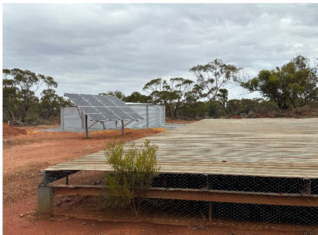
Gutha concrete lined dam roofed (Sept 2021)
