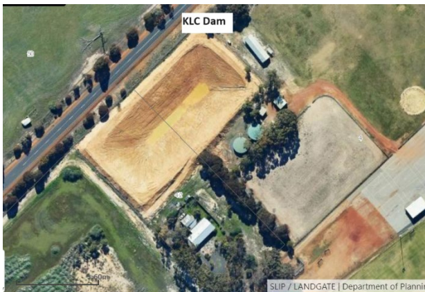
Dam at Leisure Centre
