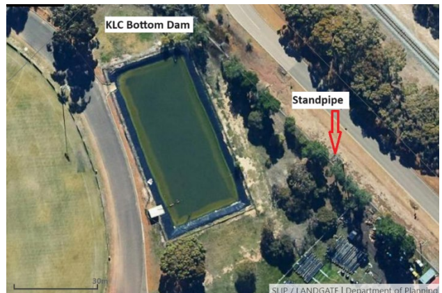
Bottom dam & standpipe at Leisure Centre
