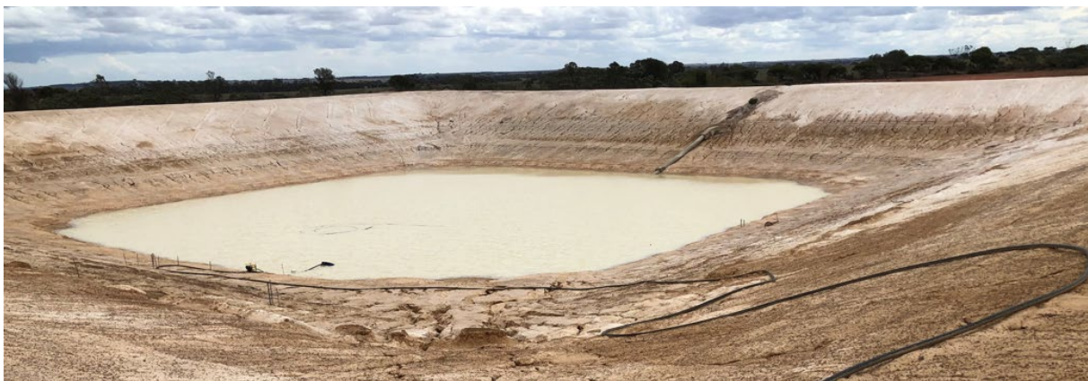
Toompup Dam (March 2020)
