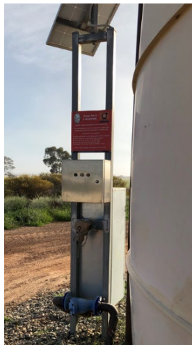
Swipe card standpipe system
