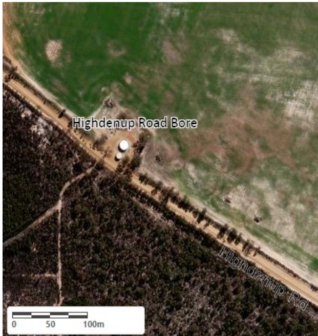
Aerial view of Highdenup Road bore
