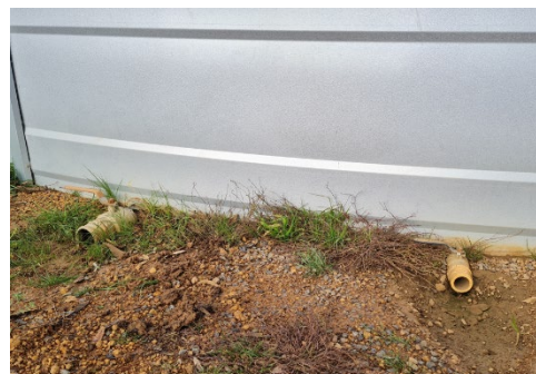
Concrete tank couplings
