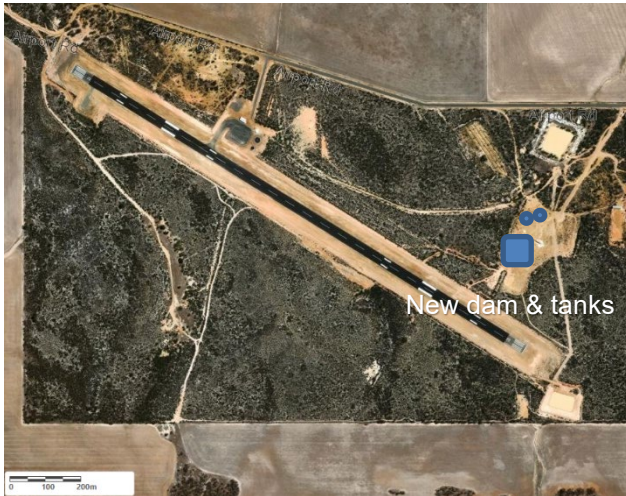
Aerial of Gnowangerup Airport Dam
