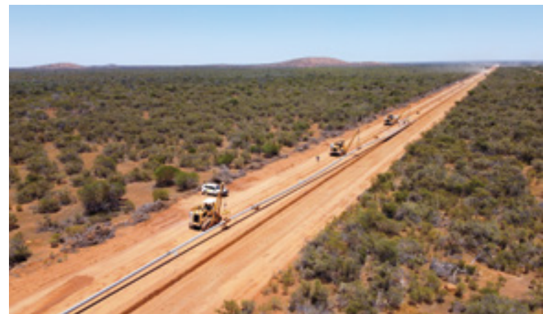
The Northern Goldfields Interconnect (gas) Pipeline
