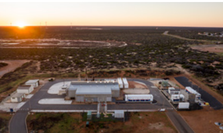
Denham power station and the renewable hydrogen microgrid.
