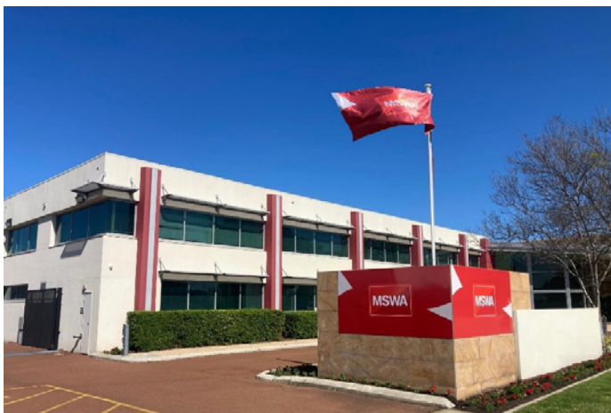
Image of MSWA Belmont, where an EV charger was installed. Image supplied by MSWA in September 2024.
