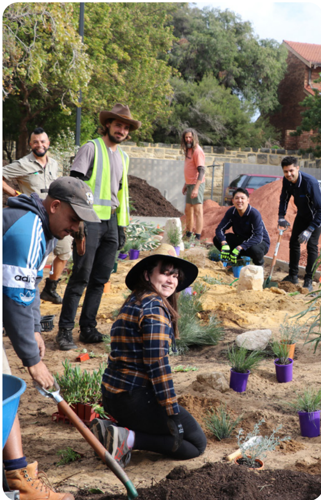
Waterwise landscaping in progress
