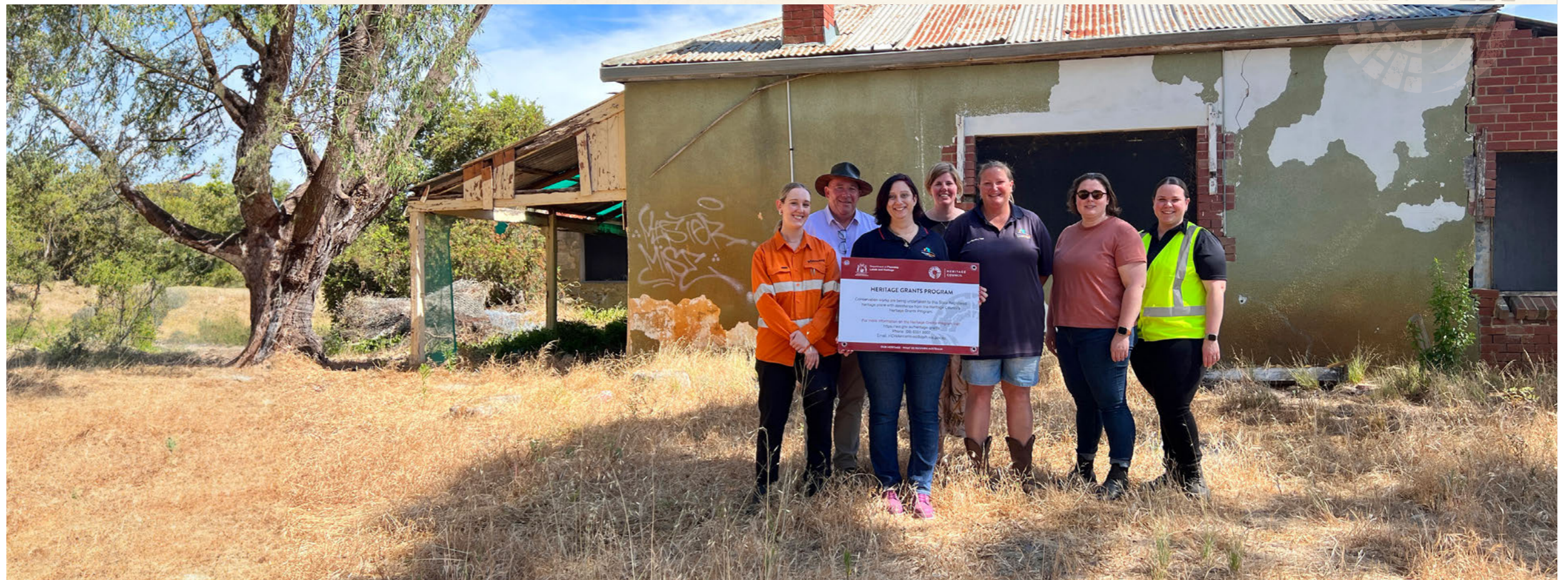
Department staff visited the Mead Homestead, Leda in December 2023 to meet the dedicated team behind the project and visit the place before the start of conservation work.
