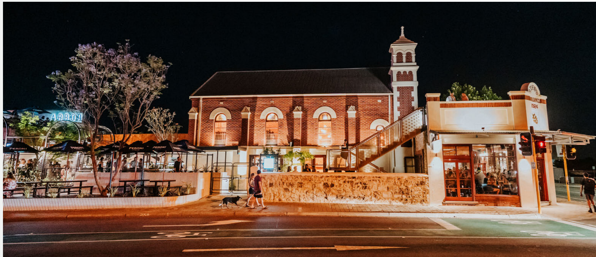
The Old Synagogue, view from Parry Street Fremantle - Kate Drennan Photography
