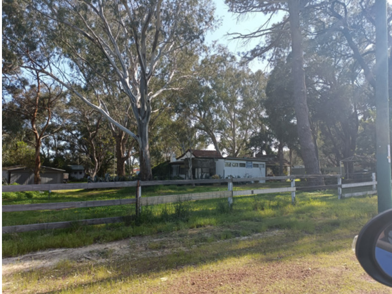
Plate 10: Built Form - Typical View Into a Rural Lot on the Subject Land Showing Various Private Buildings, Sheds and Water Tower Amongst Trees.
