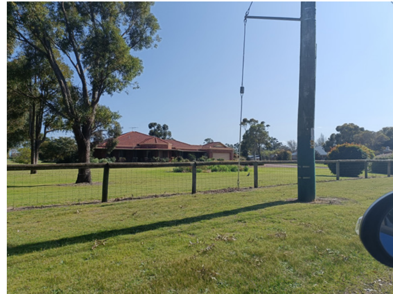
Plate 8: Built Form - Typical Large Single Storey Brick House Set Back From the Road on a Large Lot.
