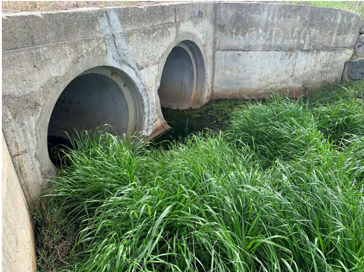
Plate 1: Discharge 1 culvert (Sept 12, 2022)
