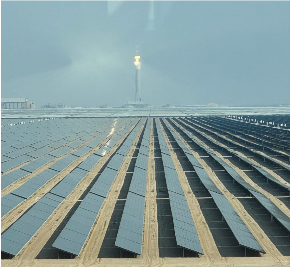
Figure 1. Mohammed bin Rashid Al Maktoum Solar Park featuring the Concentrated Solar Power (CSP) project
