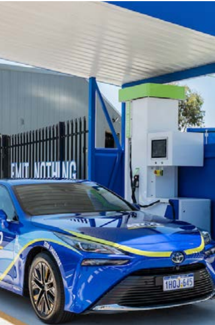
Hydrogen Refueller, Jandakot, Western Australia. CREDIT: ATCO
