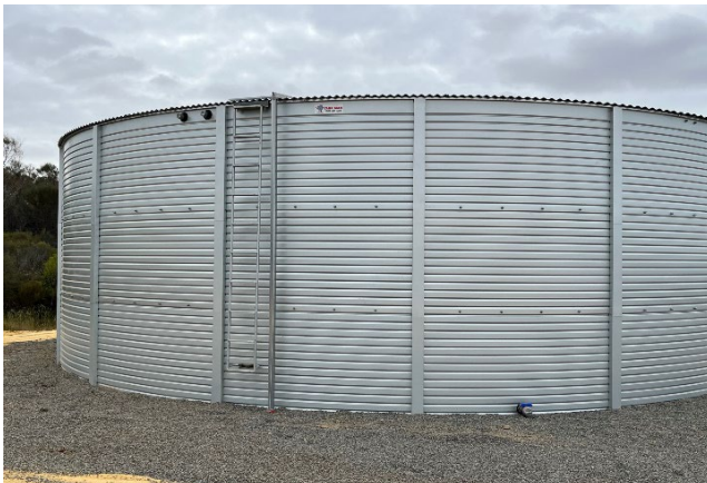
Access ladder and outlet
