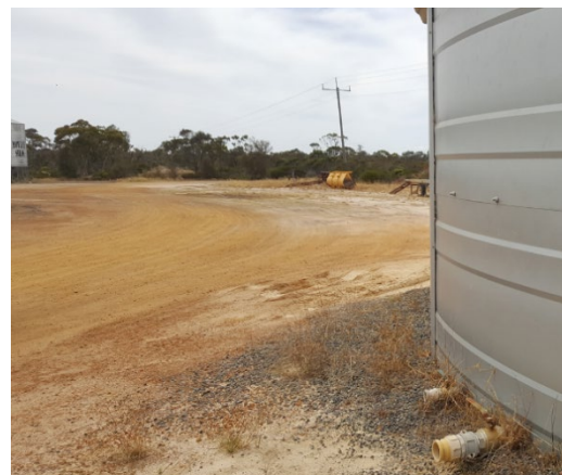
Jacup tank, access to tank camlock couplings
