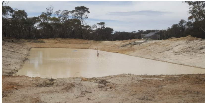
Needilup Siding Dam, solar panel and pump in distance on right bank (October 2020)
