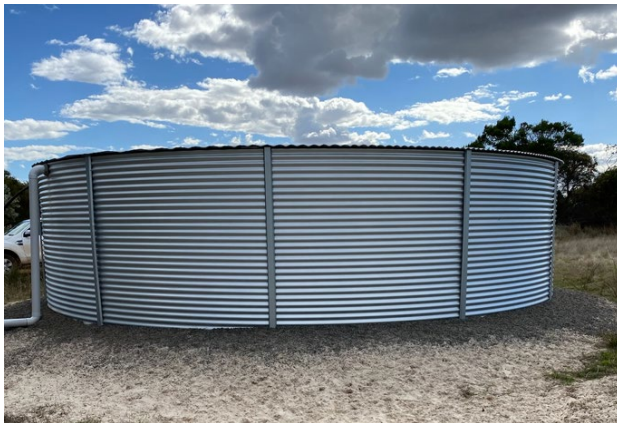
Tank 132 kL at Millers Point
