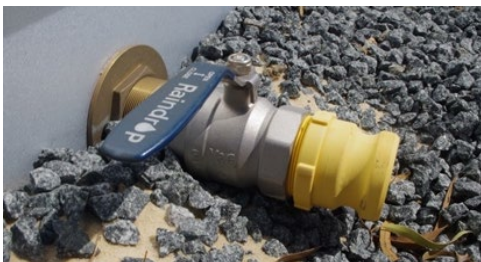
Tank standard camlock fitting
