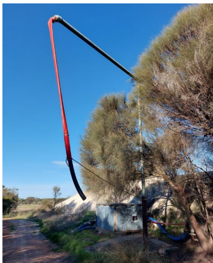
Standpipe at Houston's Dam
