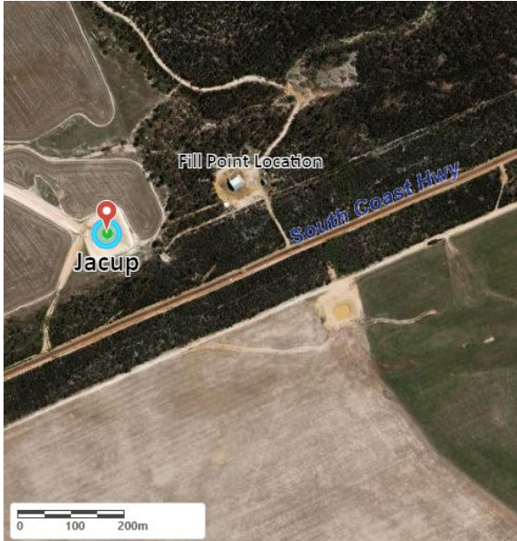
Aerial view of Jacup Dam
