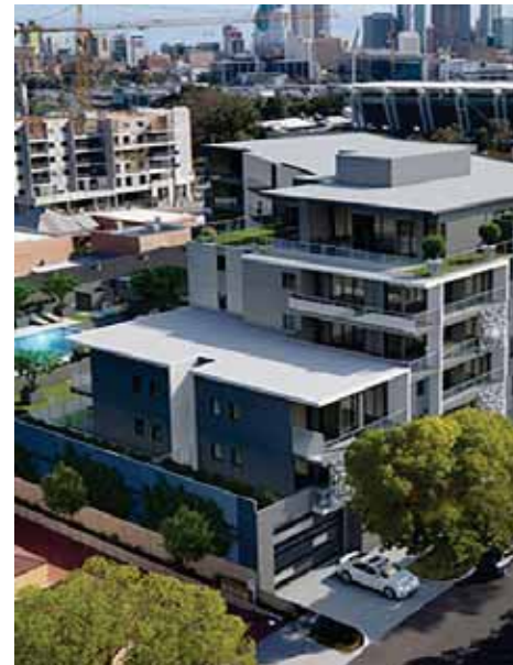
Image: Building above podium setbacks to achieve appropriate solar amenity to adjoining site
