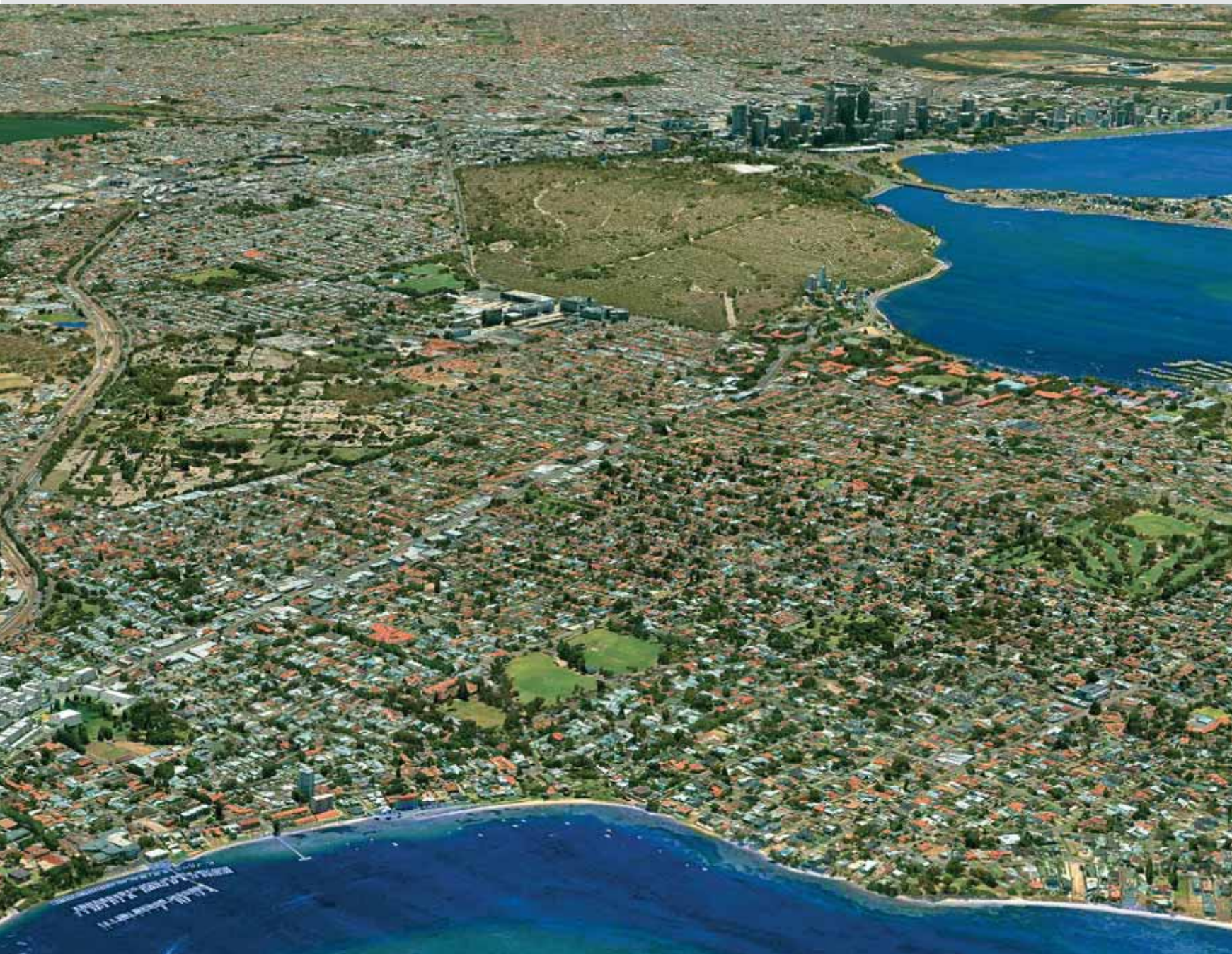
Image: Oblique view north east across the subject area, noting proximity to the Swan River and Perth CBD
