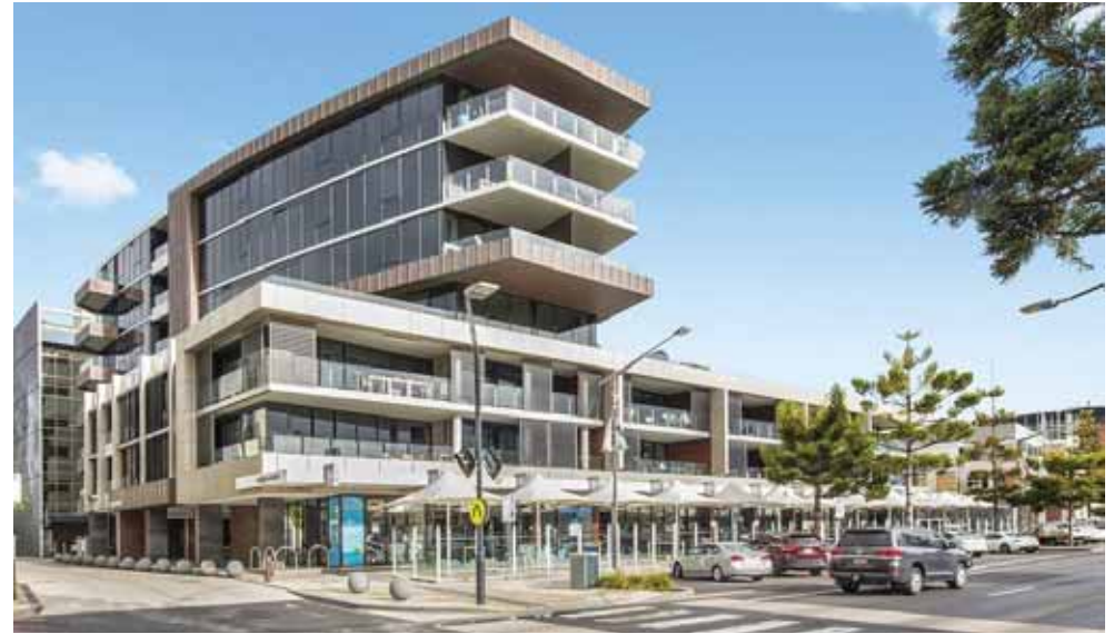
Image: Building envelopes will provide sufficient space to achieve design articulation for unique design responses
