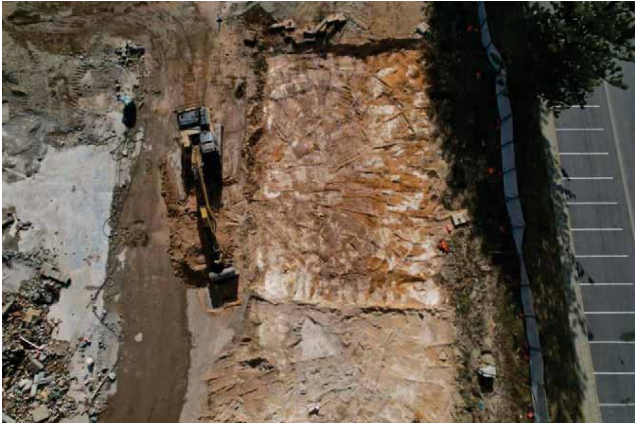
Inline Image 1: Supplied Photograph Showing Excavation of Northeast Corner
