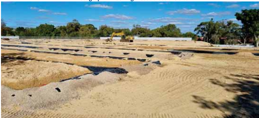
Photograph 2: Looking northeast across the site (demolished building footprints shown)
