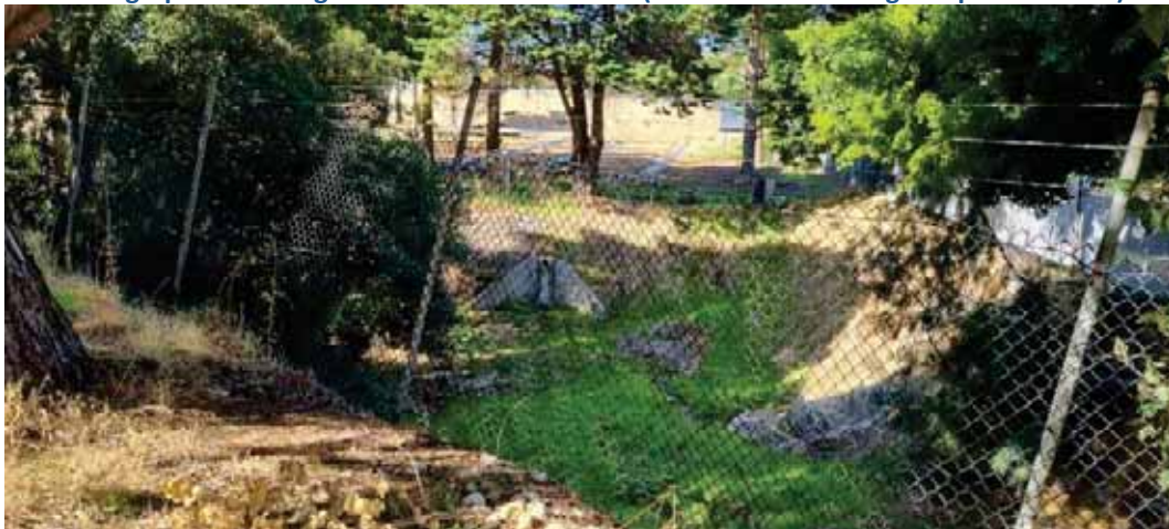
Photograph 3: Looking north at existing drainage area at the south of the site
