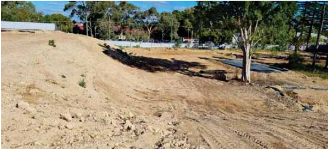
Photograph 4: Looking at existing batter near the south of the site
