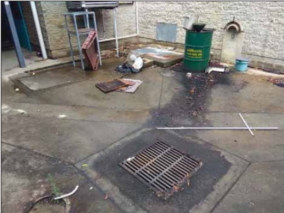
Plate 4: Fat and cooking oil storage drum, spilt fats and cooking oils on the ground surface toward a stormwater drain to the north of Building F.
