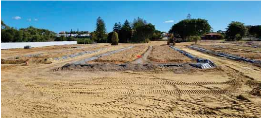
Photograph 1: Looking west across the site
