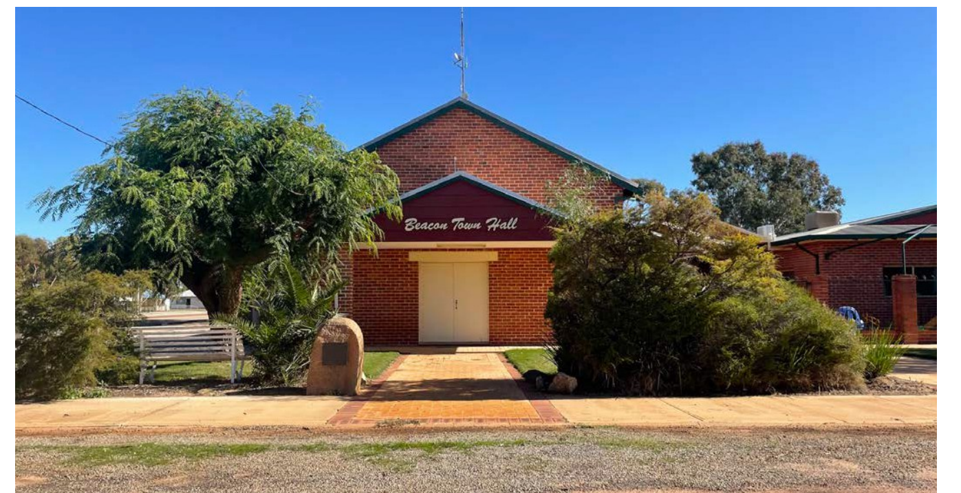
Figure 21: The Beacon Town Hall
