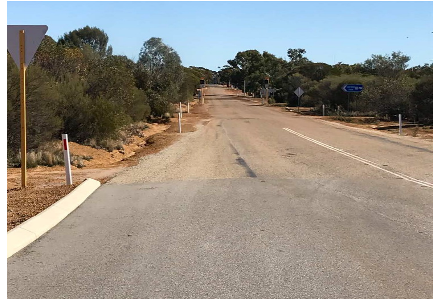
Figure 20: Beacon Road Condition
