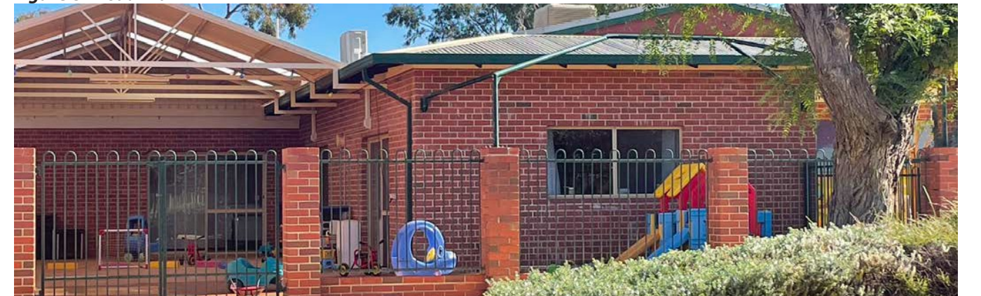
Figure 9: Beacon Daycare Facility
