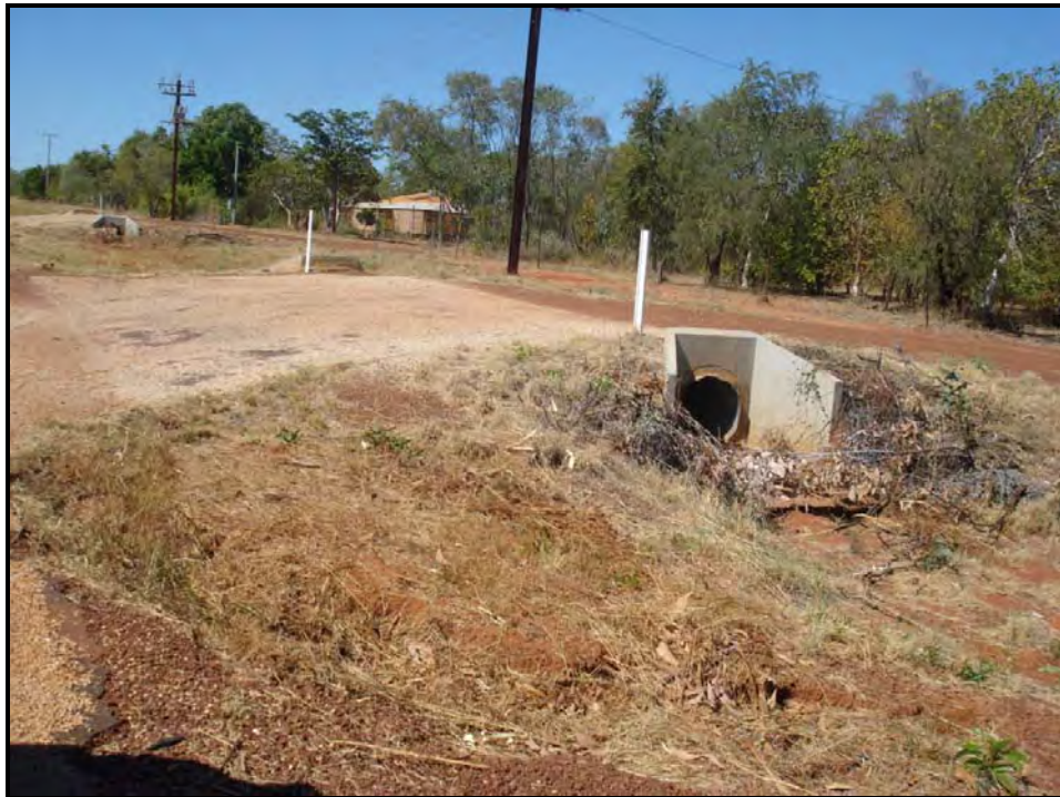
Plate 4 – Culverts under crossover along Guildford Street
