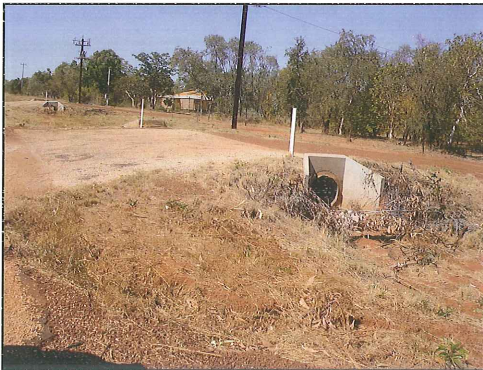
Plate 4 - Culverts under crossover along Guildford Street
