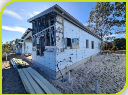
Steel frame dwellings constructed onsite on concrete slabs. Dwelling product is deemed transportable, and compliant with Residential Parks Act with regard to removable.
