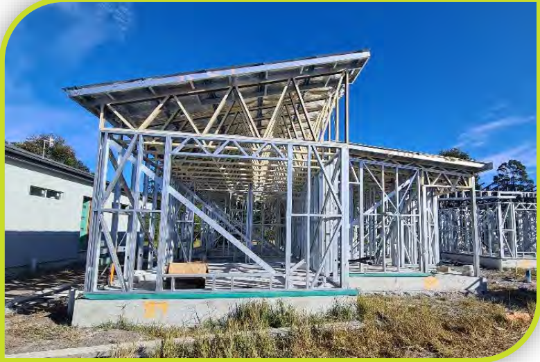
Steel frame dwellings constructed onsite on concrete slabs. Dwelling product is deemed transportable, and compliant with Residential Parks Act with regard to removable.
