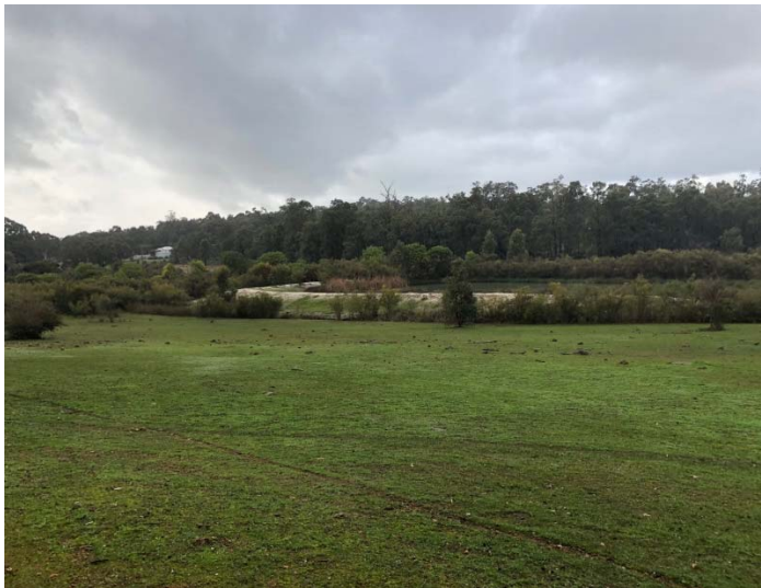
Photo 6: View of dam to the north-east looking across Parkerville 07
