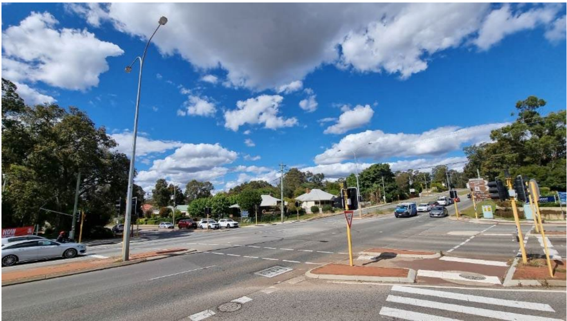
Figure 7: Great Eastern Highway/Stoneville Road/Mundaring Weir Road Intersection
