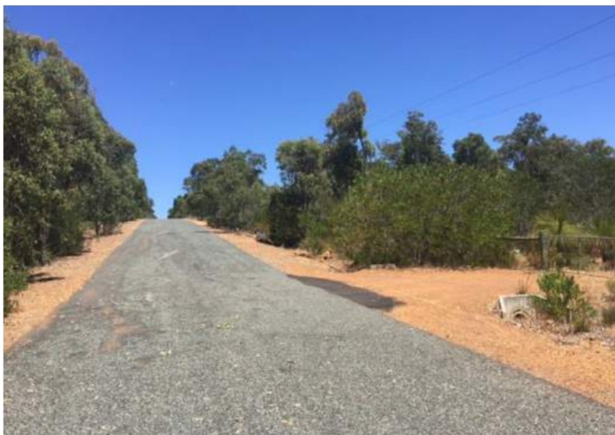
Figure 12: Existing Hawkstone Street
