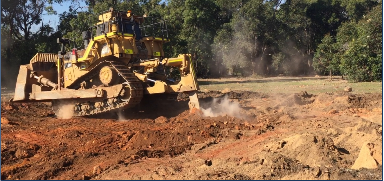
Figure 6: CAT D9T Bulldozer carrying out tipping trials
