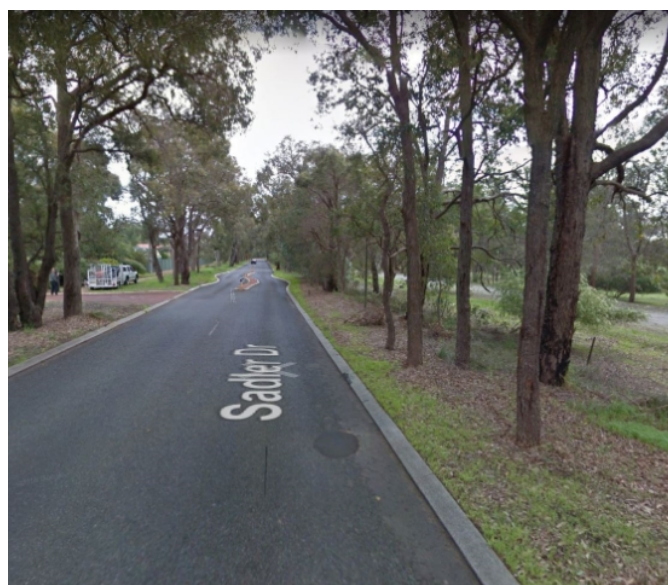
Figure 15 : Example of non-standard verge grades to facilitate tree retention
