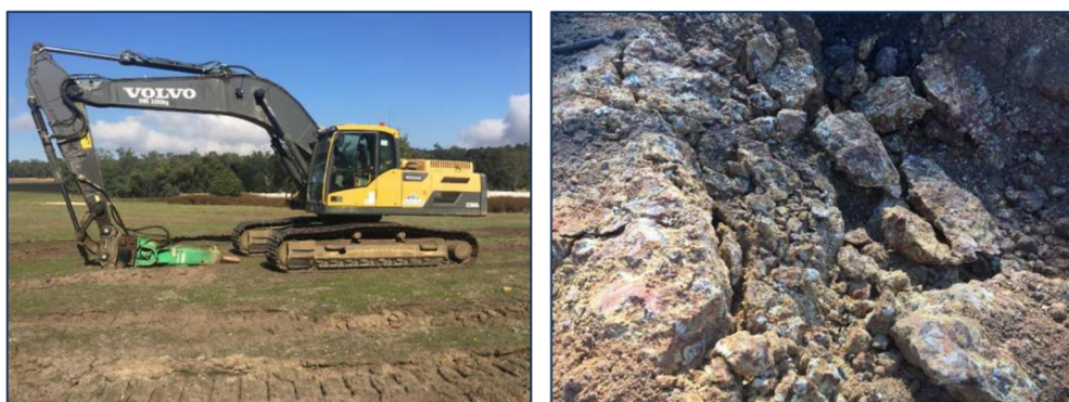
Figure 5 28T tracked excavator with rock breaking attachment (left). Hardpan Laterite (right)
