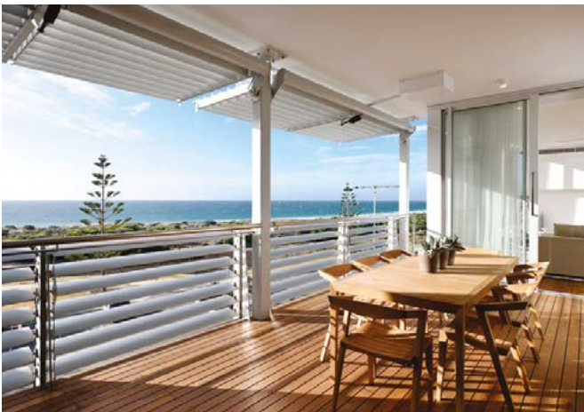
Photo 4.1c Louvred balustrades and operable awnings allow residents to adapt the balcony for light or shade throughout the day, as well as controlling shelter and privacy. (PC)
