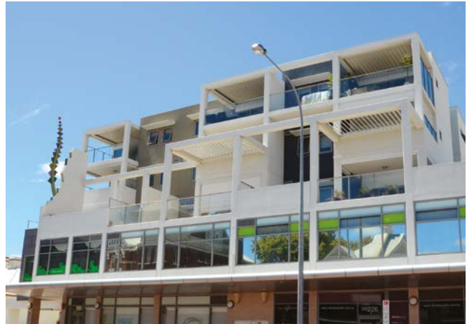
Photo 4.1d Shading and glare-control measures help to moderate solar gain for west-facing windows and balconies, including operable roof louvers to optimise sunlight and shelter.
