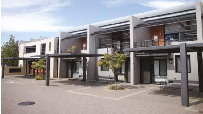
Photo 3.9a Open carport structures offer shade and shelter while maintaining good sightlines.
