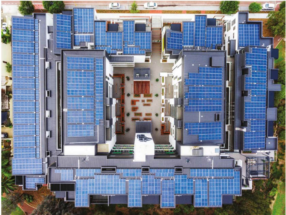
Photo 4.15a This apartment development fully utilises the roof with the installation of photo-voltaic arrays to supplement the power consumption of the dwelling units. (PC)
