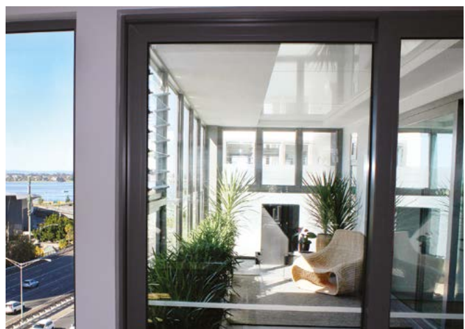
Photo 4.7c Sliding sash glazing and louvre windows in this wintergarden enables modulation of enclosure and openness, at the same time reduces the impact of traffic noise from the adjacent freeway. Installation of special noise absorbing ceiling material also helps in noise reduction.
