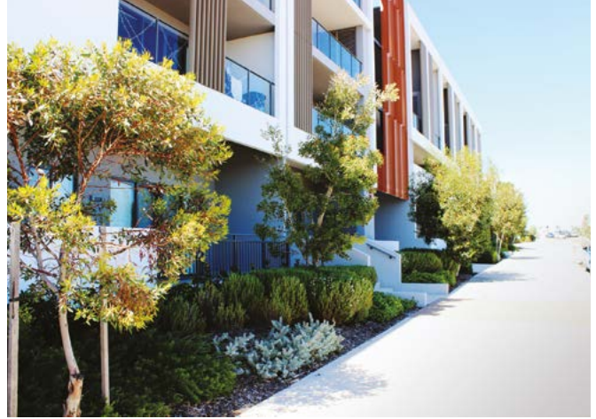
Photo 4.12d Planting between dwellings and public footpath provides a soft and attractive interface.
