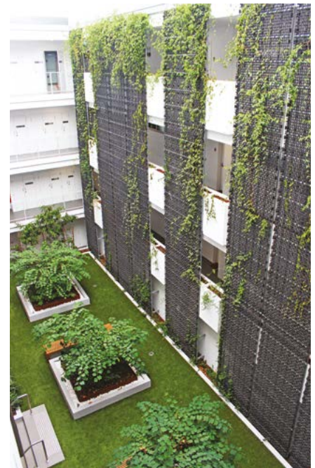
Photo 4.12b Planting along internal courtyard walls can help create a shaded, attractive space.
