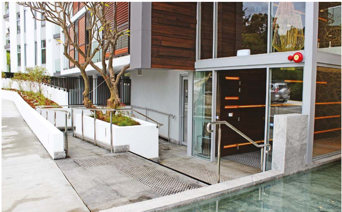
Photo 4.9a A step-free entrance is provided in this apartment block, taking into consideration universal access.
