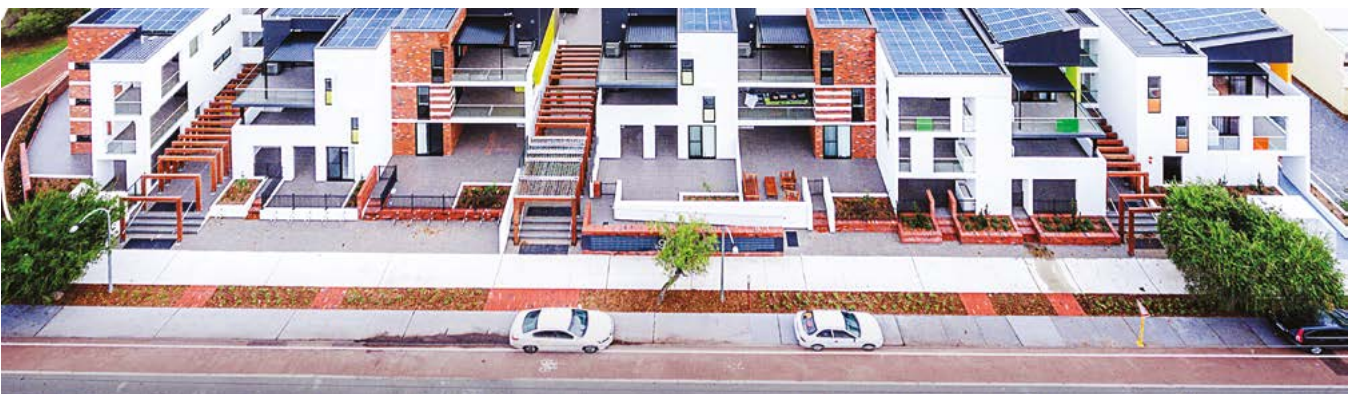
Photo 3.6h Some good public interface elements are demonstrated here: the three street entry points are clearly legible, one of them has universal access; change in level between footpath and front courtyards for privacy allowing for largely permeable fencing; upper level balconies and windows overlook the street and public domain areas ensure public surveillance; mix of textures and materials provide pedestrian interest; mail boxes and bike racks are well integrated along front fences; landscaping provision is generous and enhances the layout design. (PC)
