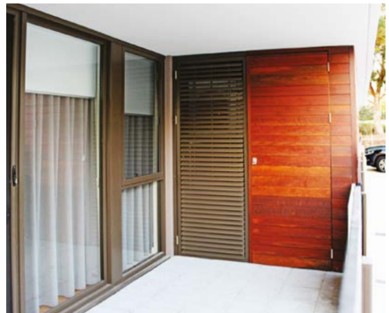
Photo 4.6b This storage area is integrated into the balcony design, weatherproof and screened from view.
