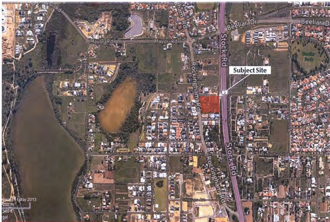
Figure 1. Aerial photo of the subject site
