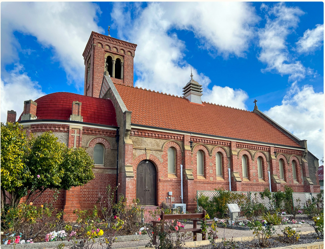
ABOVE: All Saints' Anglican Church, Collie P552 2021-22 SHG recipient for Conservation Management Plan and works to the belfry.
