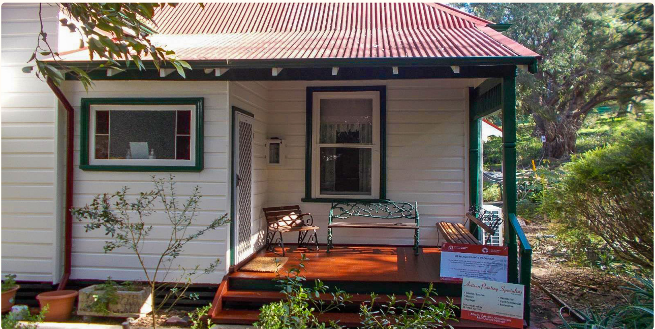
ABOVE: Tom Collins House, Allen Park P2368
