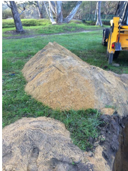
TP05 – TEST PIT EXCAVATION
