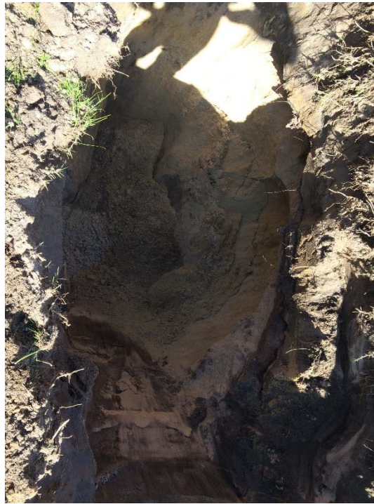
TP08 – TEST PIT EXCAVATION
