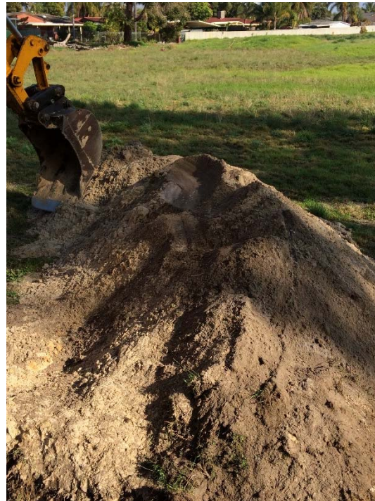
TP08 – TEST PIT EXCAVATION
