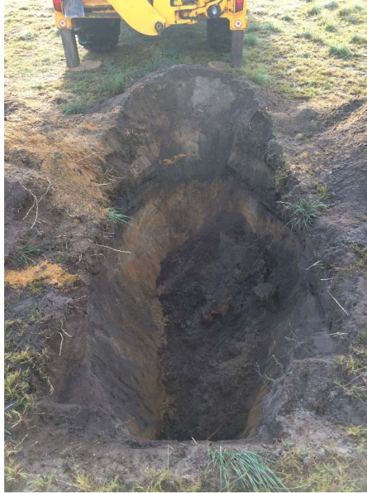
TP03 – TEST PIT EXCAVATION
