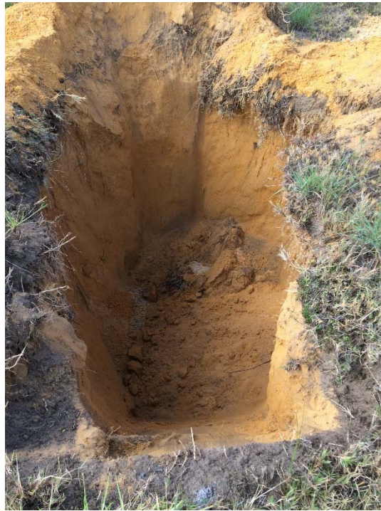
TP12 – TEST PIT EXCAVATION
