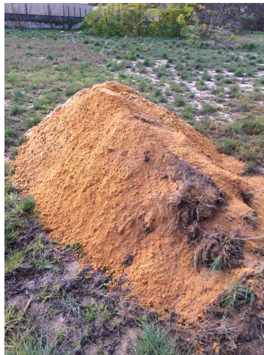
TP12 – TEST PIT EXCAVATION
