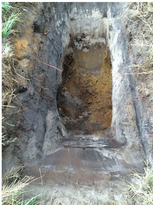
TP10 – TEST PIT EXCAVATION
