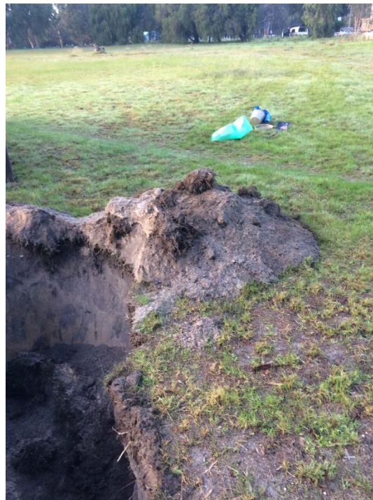
TP02 – TEST PIT EXCAVATION
