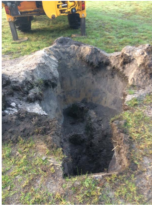
TP02 – TEST PIT EXCAVATION
