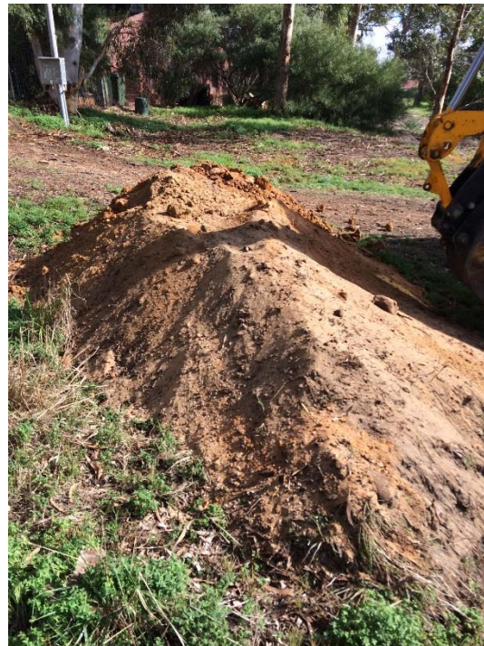
TP09 – TEST PIT EXCAVATION
