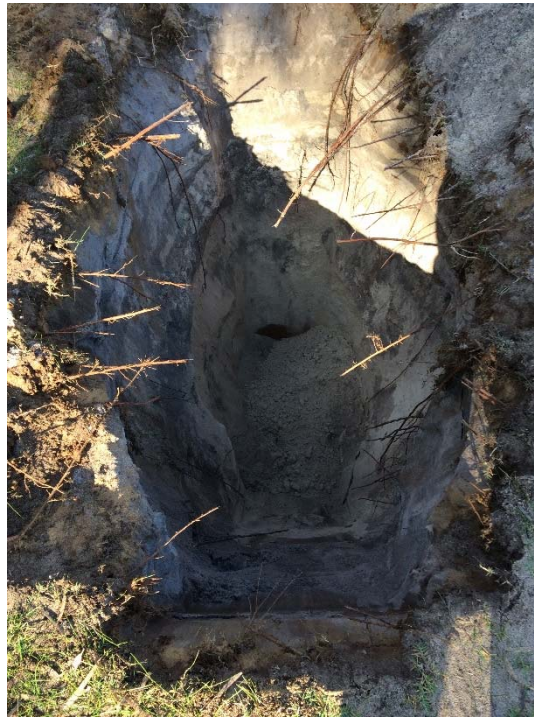
TP06 – TEST PIT EXCAVATION
