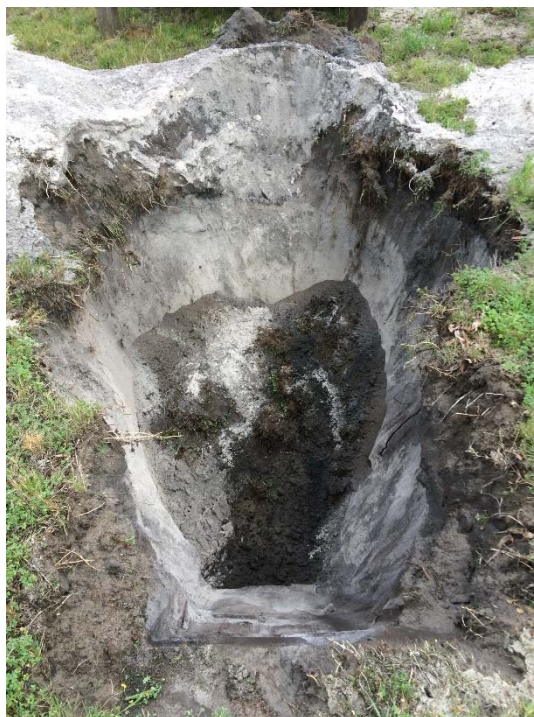
TP11 – TEST PIT EXCAVATION
