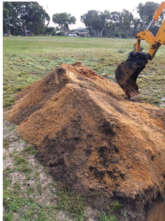
TP04 – TEST PIT EXCAVATION
