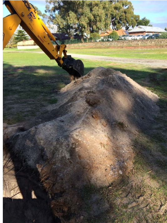
TP06 – TEST PIT EXCAVATION
