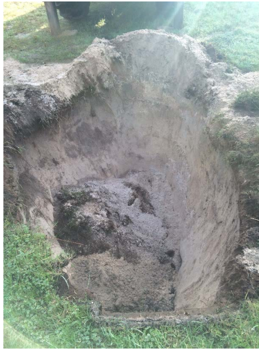
TP01 – TEST PIT EXCAVATION
