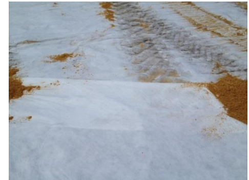
Photograph 6. Geotextile warning barrier
