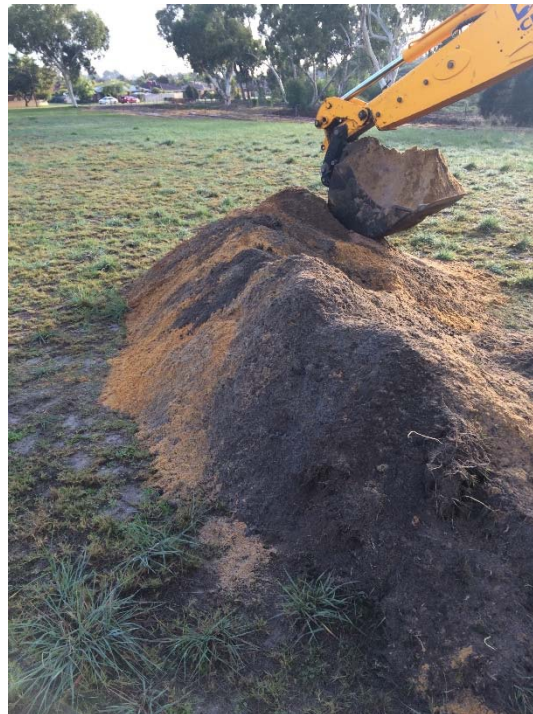
TP03 – TEST PIT EXCAVATION
