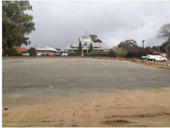
Photograph 3. Containment Cell: Road base over warning barrier Containment Cell
