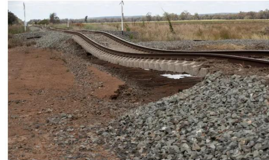
Flood damage on the Parkes-Condobolin railway line in central west NSW. Photograph: Mike Bowers/The Guardian
