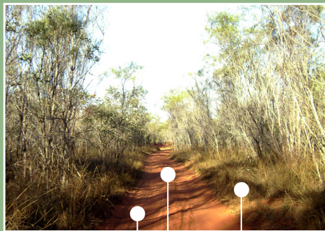
Unsealed surface | Narrow lane width | Unkerbed, vegetated edges
