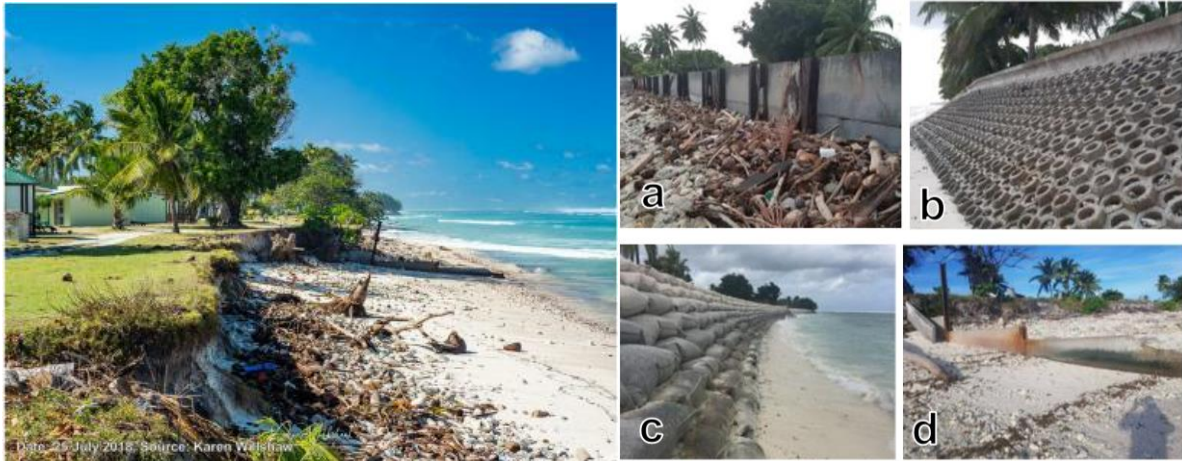
Figure 75: Recent erosion along unprotected West Island settlement shoreline (left) and on right is photographs of the series of coastal protection structures introduced to protect the West Island settlement (a) older vertical seawall (b) Seabee seawall (c) GSC revetment and (d) older groynes.
