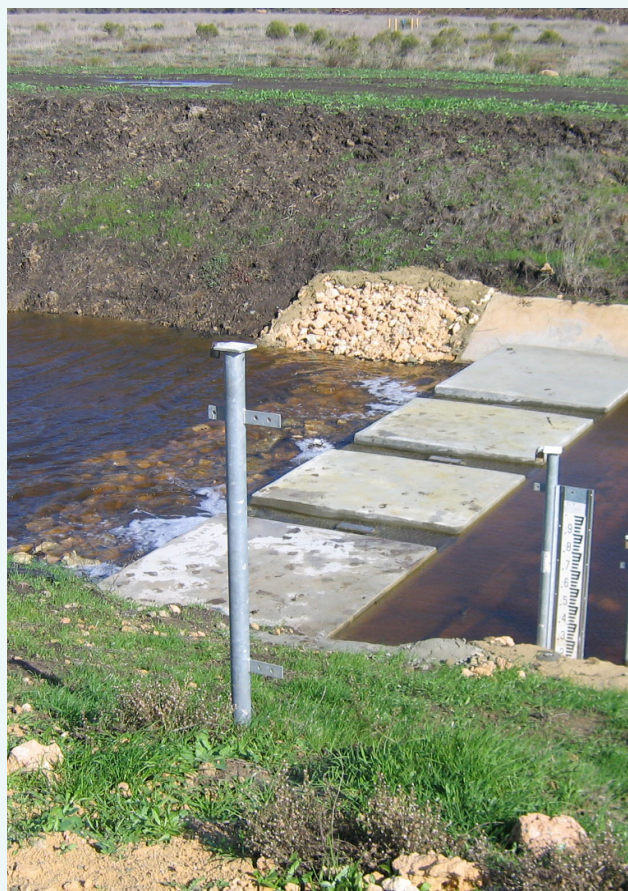
The weir at the Peel Main Drain sampling site, May 2007.
