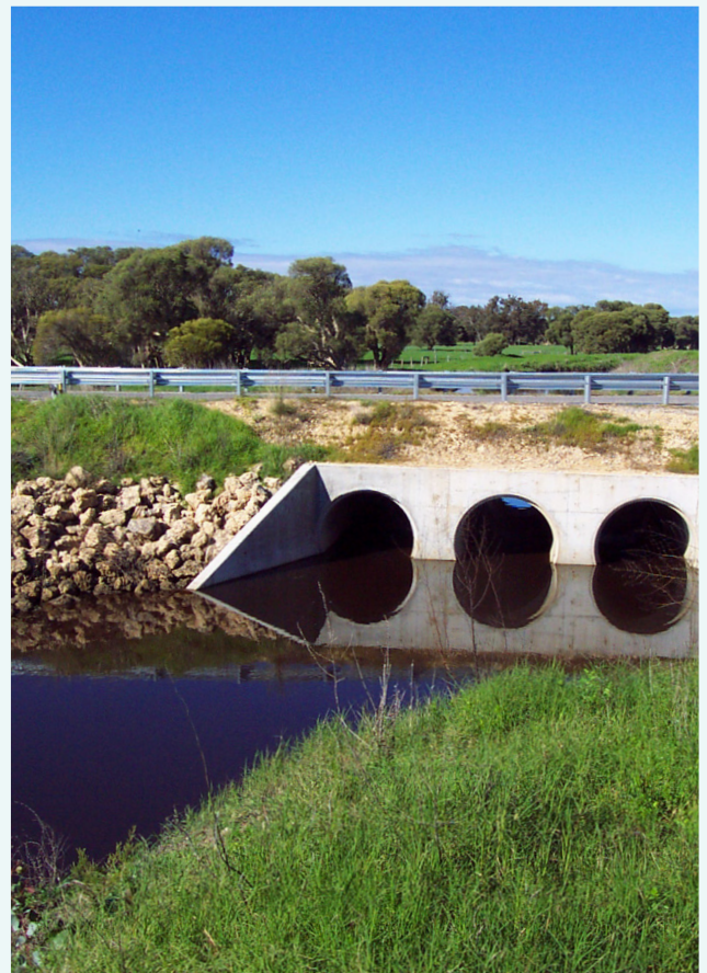
The culverts where Peel Main Drain passes under Karnup Road near the sampling site, July 2002.
