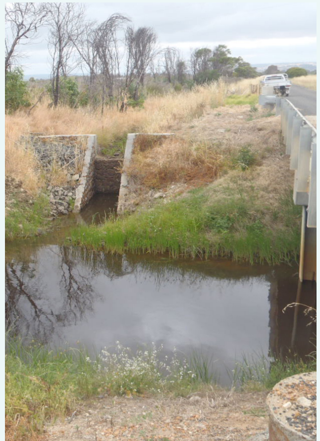
A side drain (not flowing when this picture was taken) which enters Mangosteen Drain just upstream of the sampling site at Leitch Road, December 2018.
