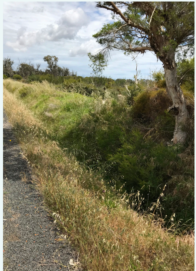
A roadside drain. These drains help to quickly transport water from the road to larger drains, November 2020.
