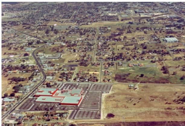
Figure 9.2: Aerial View over Westfield Carousel 1972 looking North-West
