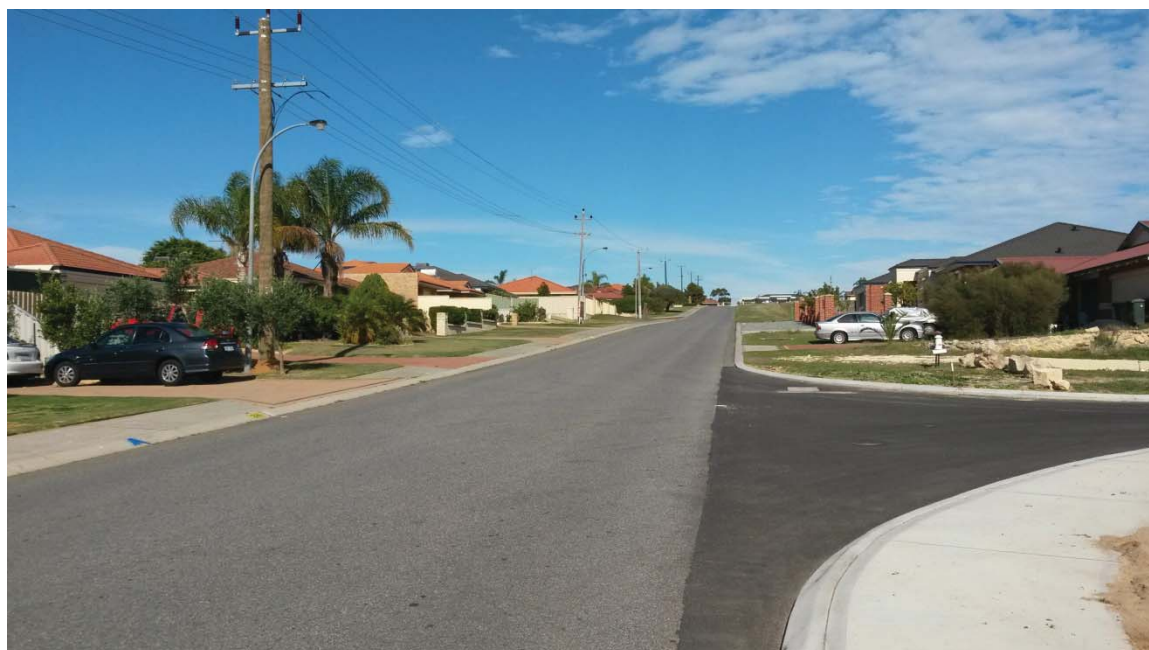
Figure 3: Southbound view along Watson Road in the vicinity of the East-West road intersection
