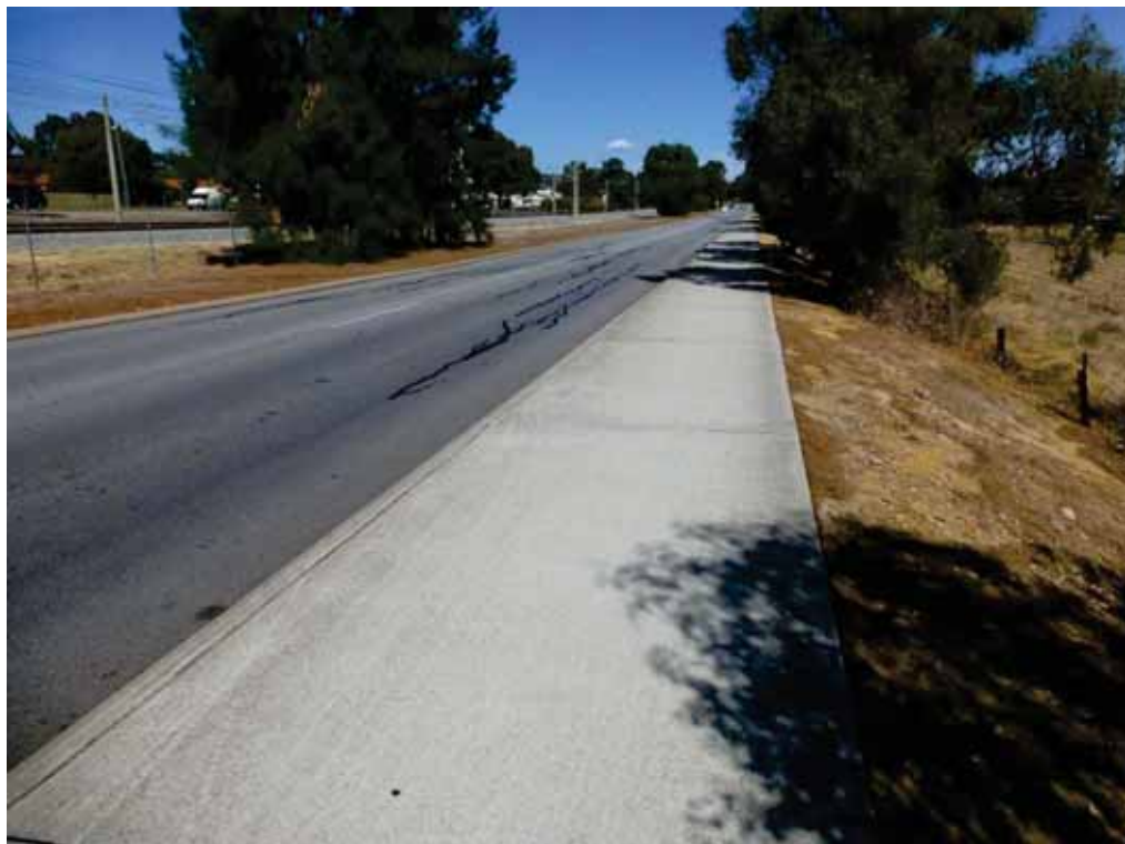
Photograph 4: Embankment along Railway Avenue (eastern boundary)
