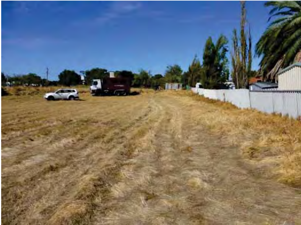
Photograph 1: Looking south – CPT rig at CPT01 location
