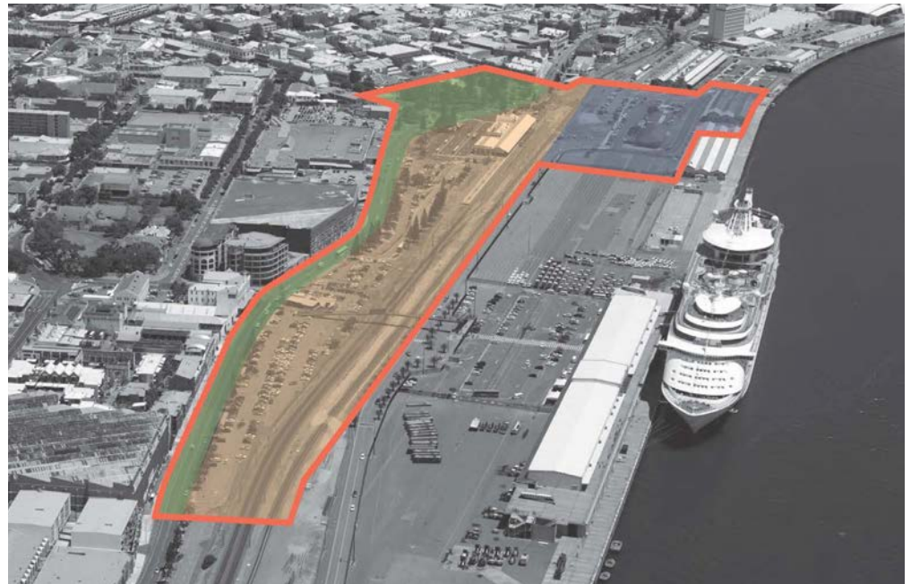
The project area containing the three precincts. Not to scale. Fremantle Railway Station and adjoining PTA land in light orange (6.4 ha)
