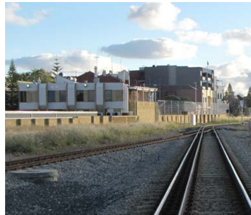
Existing pedestrian crossing environment looking southwest.
