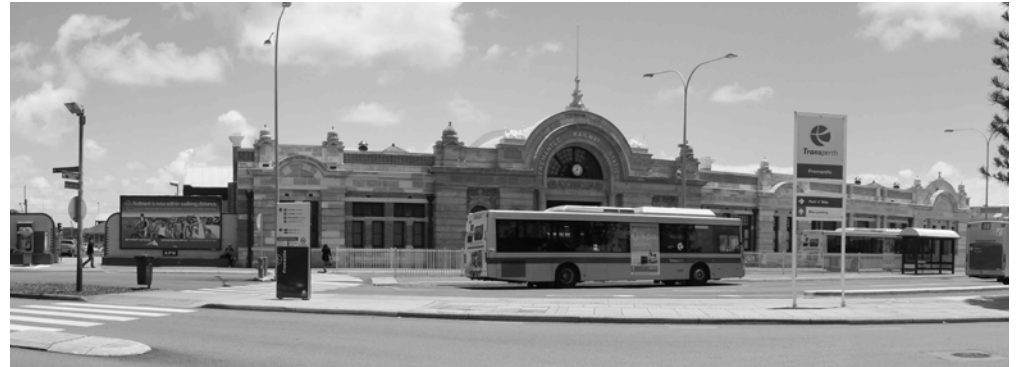
Fremantle Railway Station, showing existing bus interchange area.
