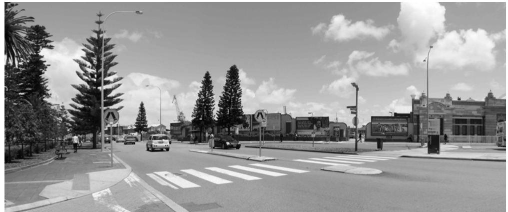
Pedestrian crossing from Fremantle Railway Station to Market Street.
