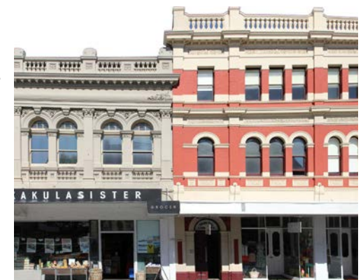
Market Street building facades.
