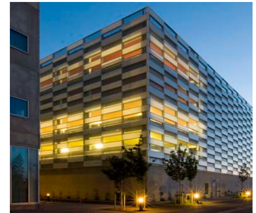
Multi-decked parking in Sweden.
