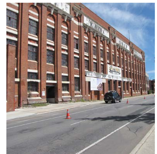
Former Woolstores building opposite railway, typical harbourside area building.
