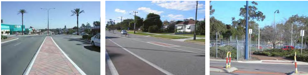
Figure 3.1 Examples of raised median, painted median and pedestrian refuge islands
