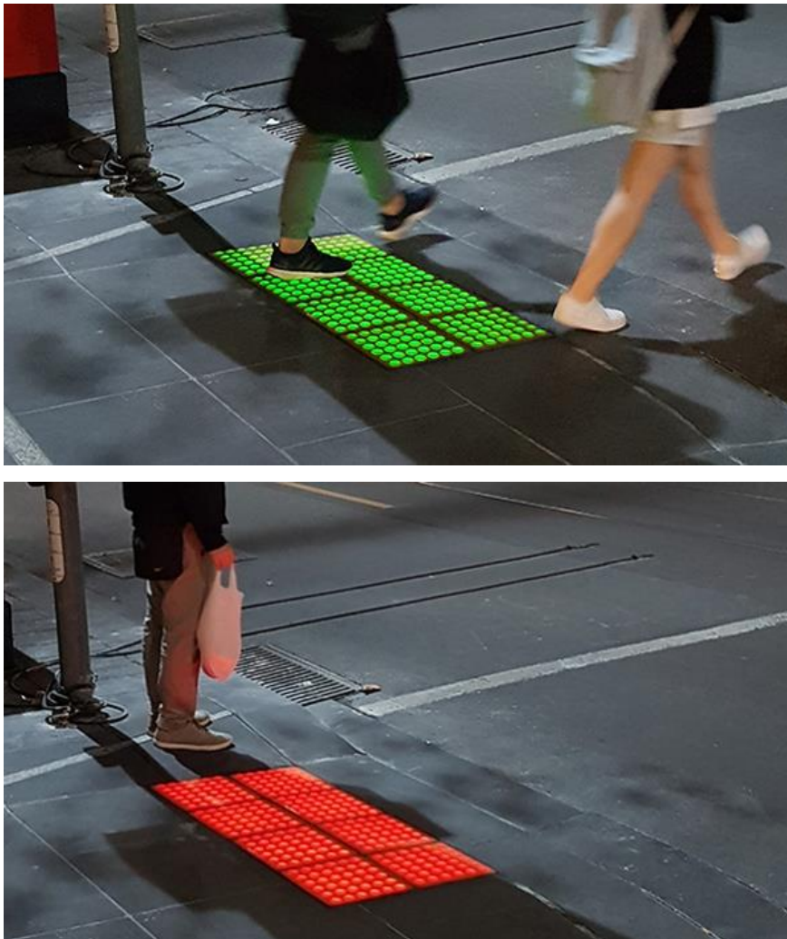
Figure 3.11 In-ground pedestrian lights in Melbourne
