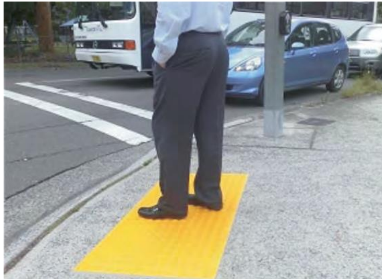
Figure 3.13 Pedestrian switch pads
