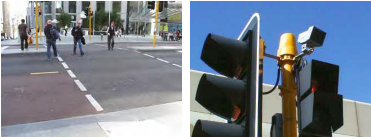
Figure 3.3 Examples of a Pelican crossing (left) and the pedestrian detector on a Puffin crossing (right)
