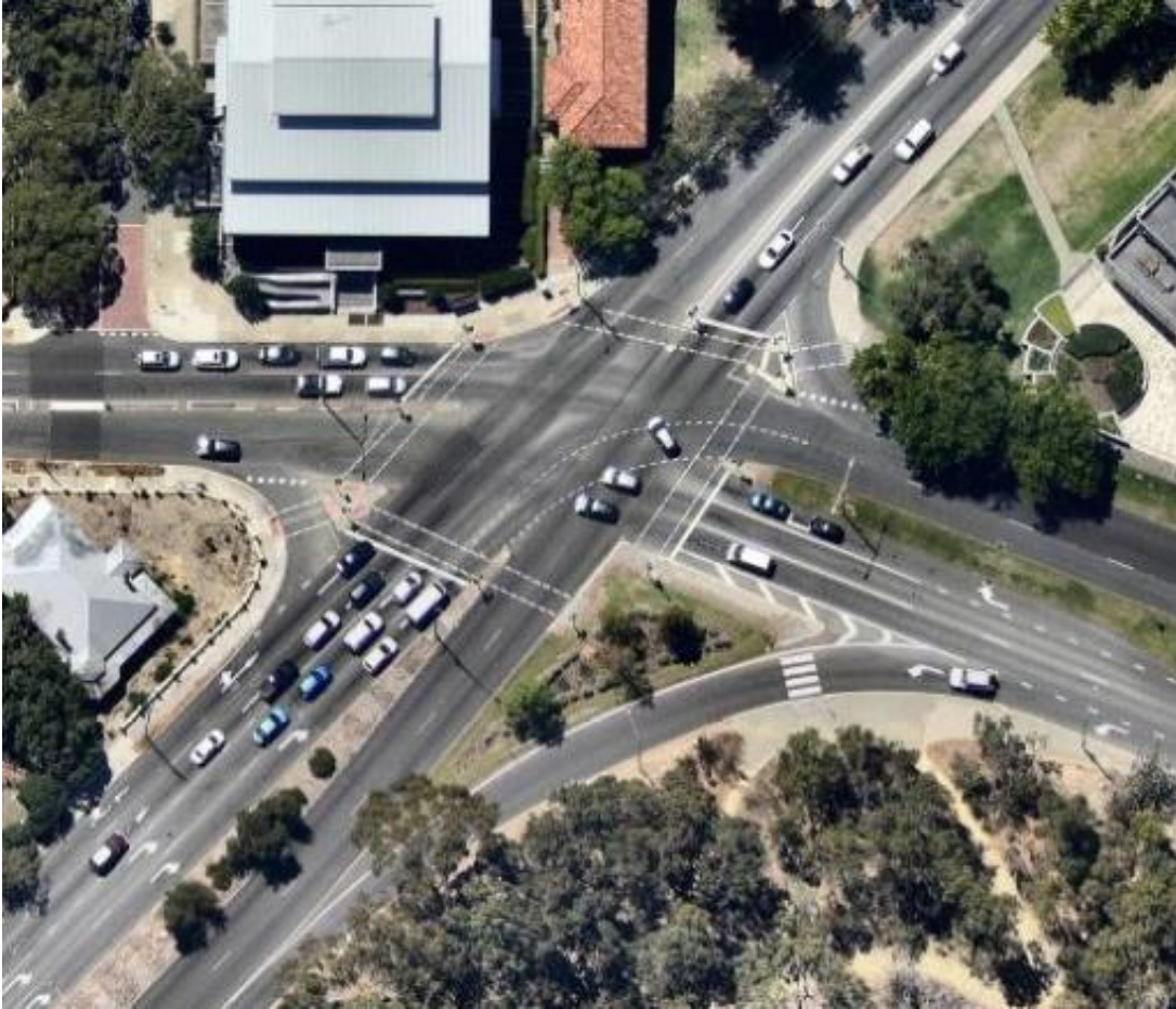
Figure 12: Thomas Street/Bagot Road and Kings Park Road, West Perth
