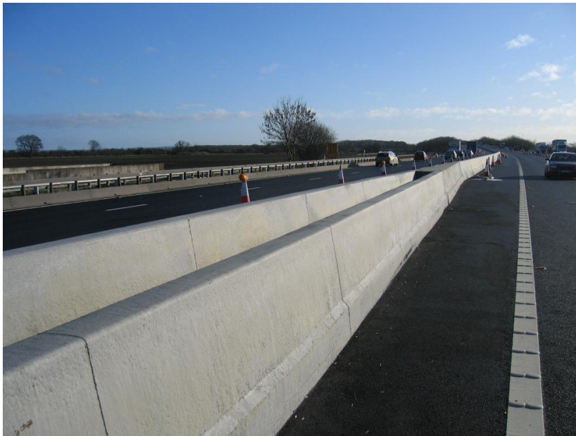
Figure 2: A concrete safety barrier
