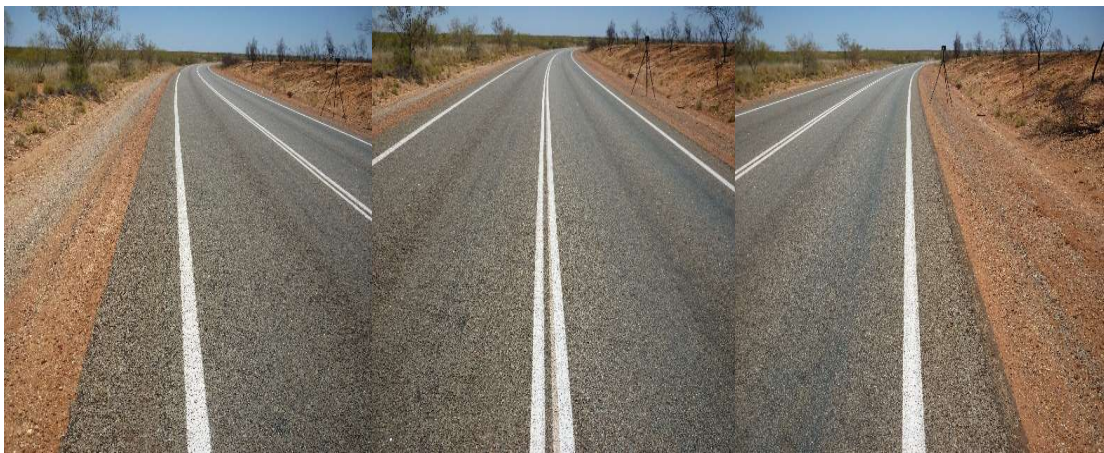
Figure 2.38 Site 16 photographs – facing southbound
