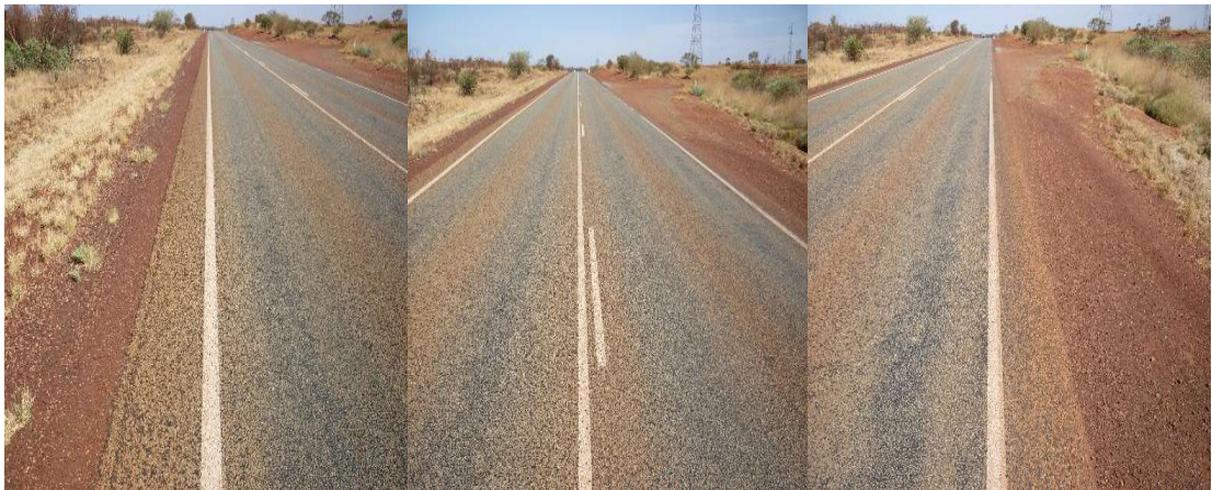
Figure 2.26 Site 10 photographs – facing southbound
