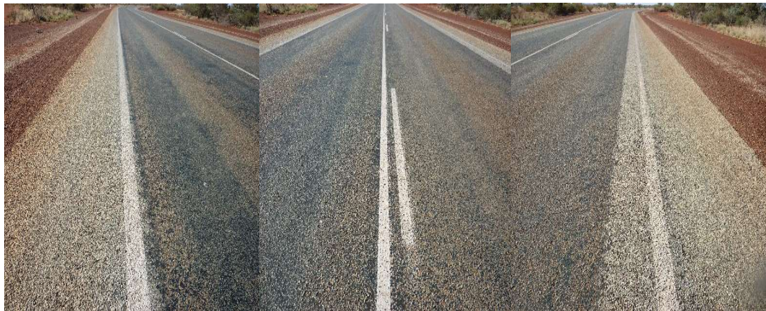
Figure 2.10 Site 2 photographs – facing northbound
