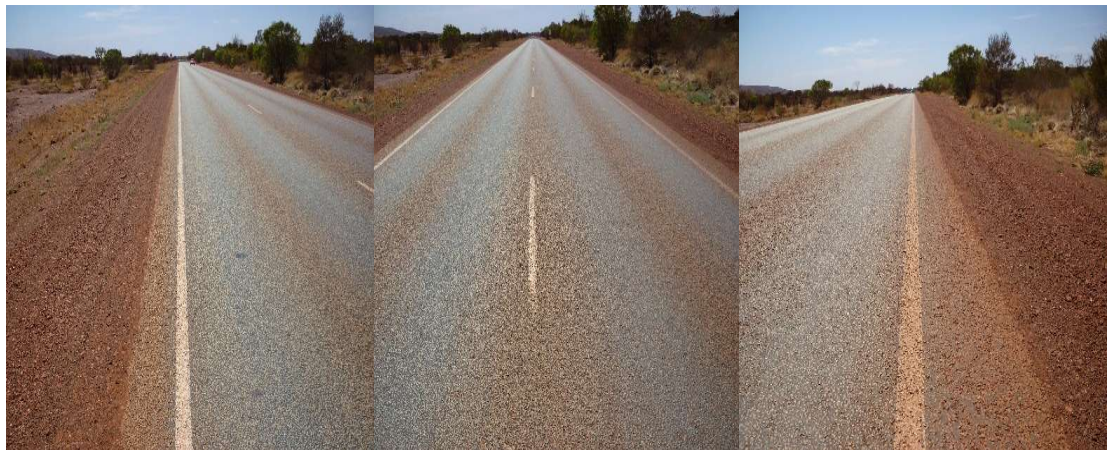
Figure 2.20 Site 7 photographs - facing southbound
