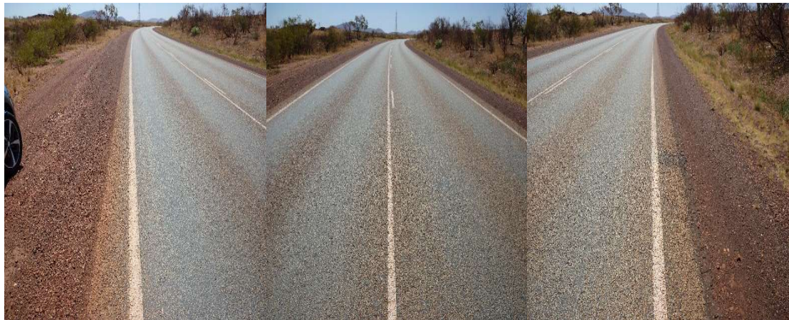
Figure 2.24 Site 9 photographs – facing northbound
