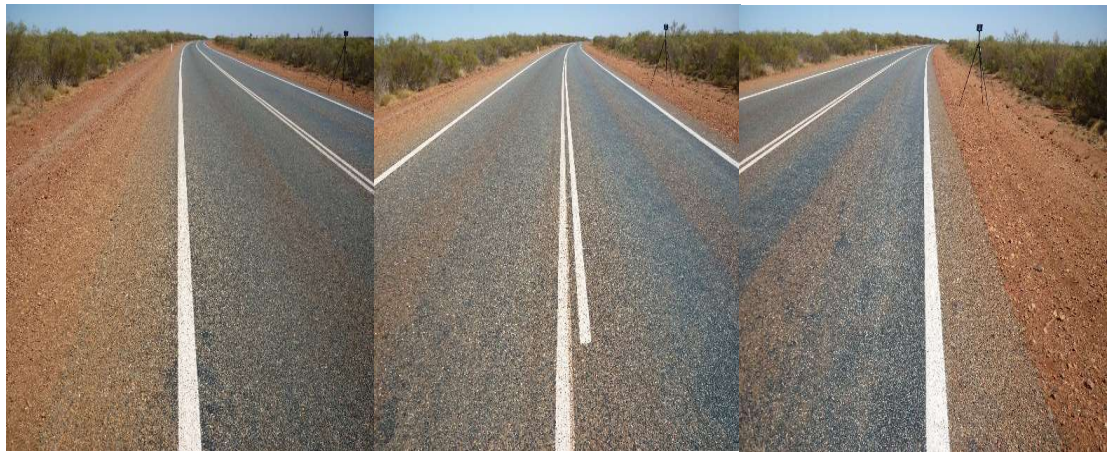
Figure 2.42 Site 18 photographs – facing southbound
