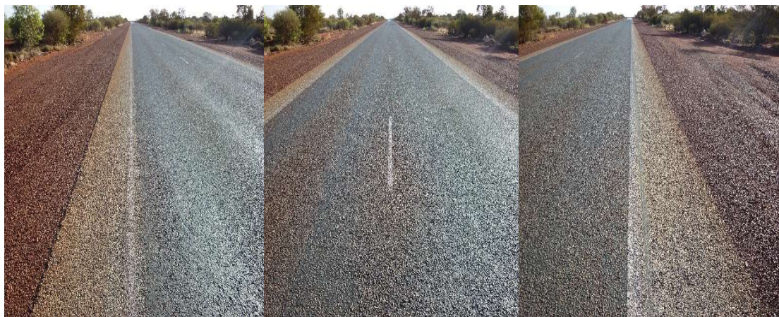
Figure 2.12 Site 3 photographs – facing northbound
