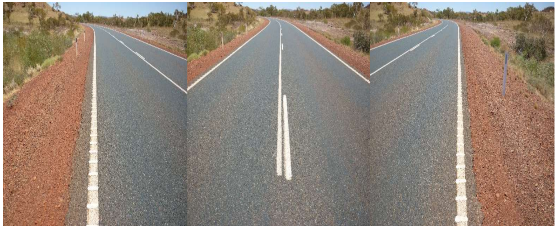
Figure 2.30 Site 12 photographs – facing northbound
