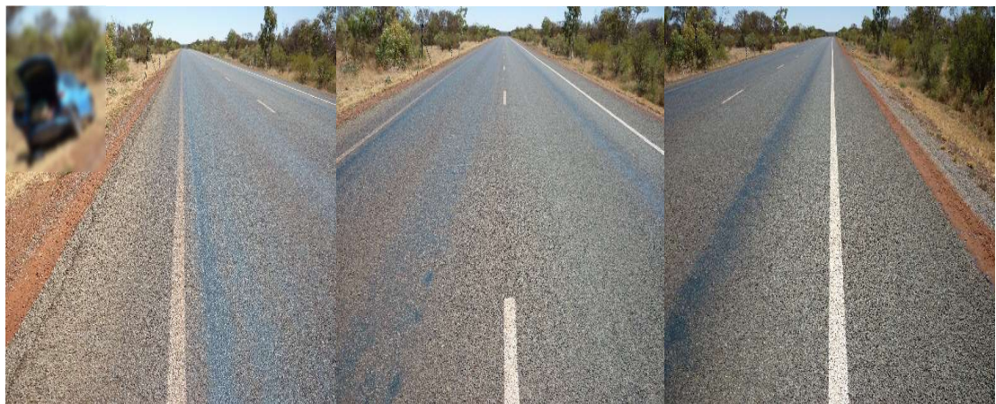
Figure 2.44 Site 19 photographs – facing southbound
