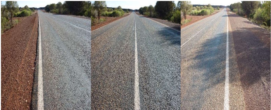
Figure 2.8 Site 1 photographs – facing southbound
