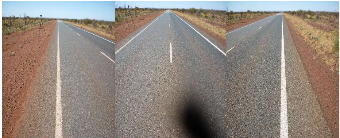
Figure 2.34 Site 14 photographs – facing southbound
