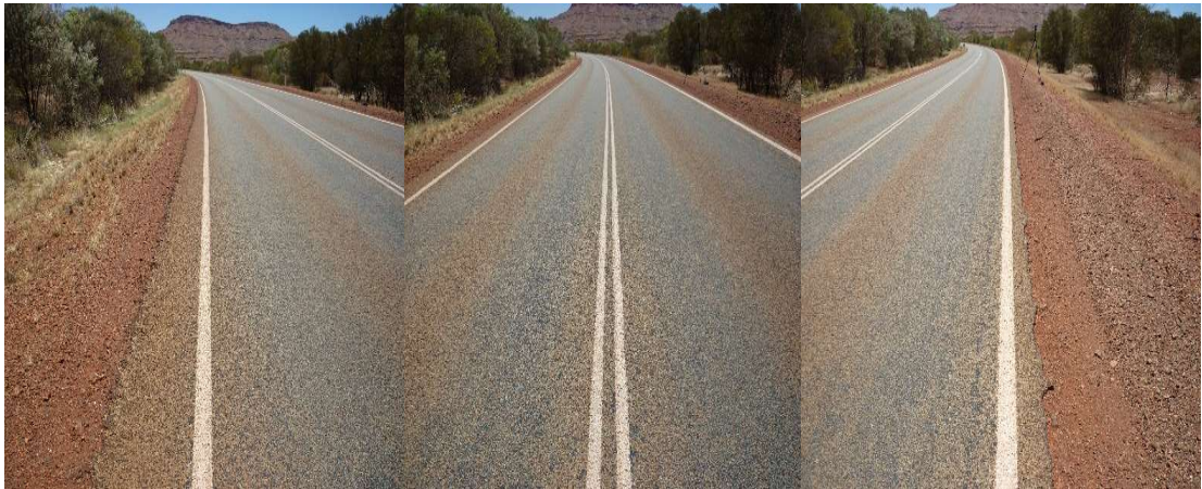
Figure 2.32 Site 13 photographs – facing southbound
