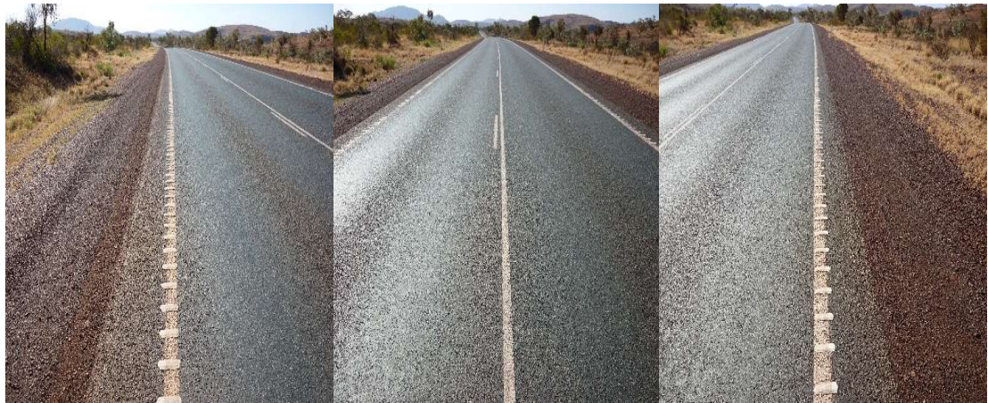
Figure 2.28 Site 11 photographs – facing southbound
