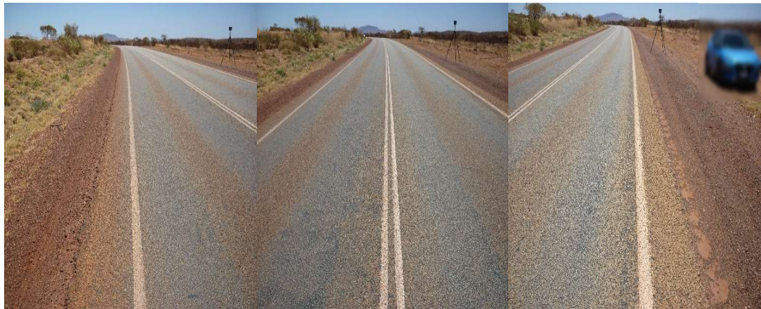
Figure 2.22 Site 8 photographs – facing southbound
