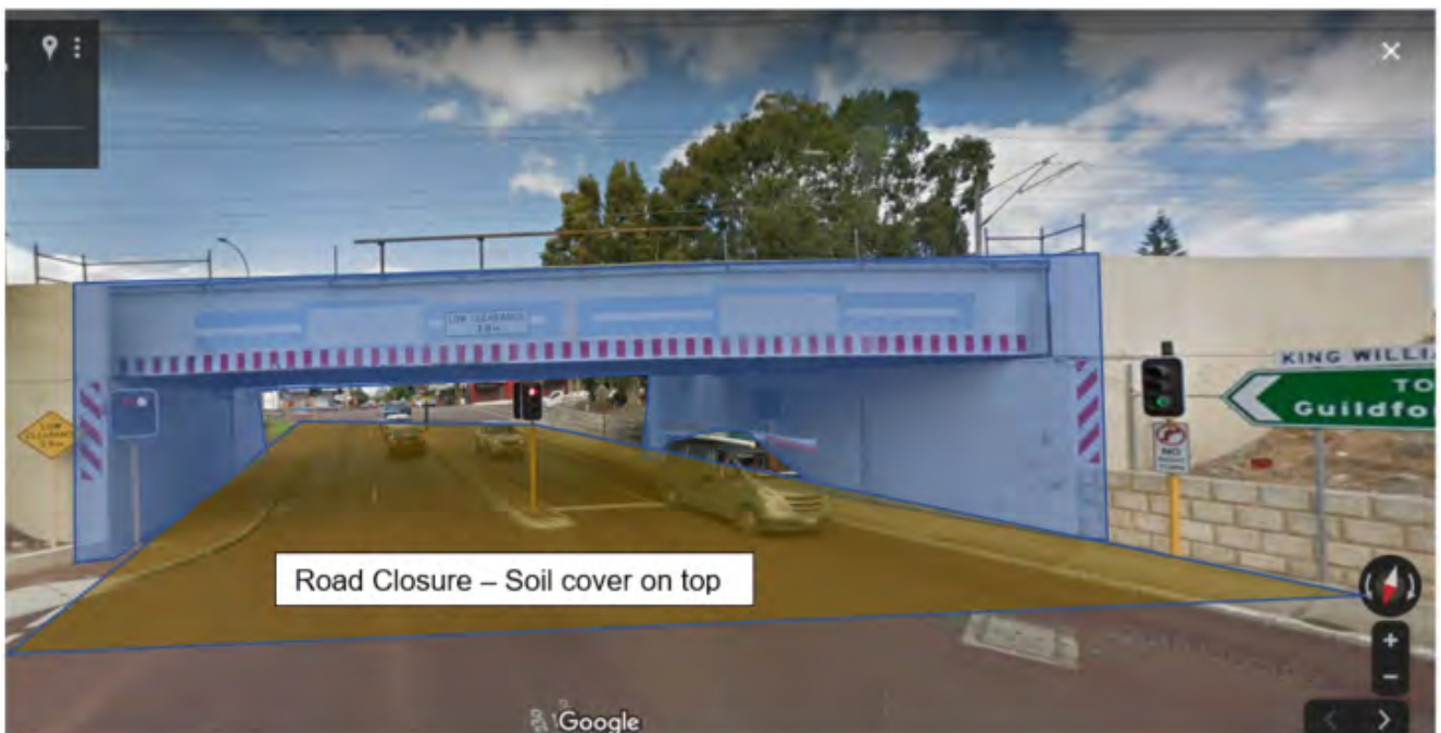
Figure 18.59: King William St. Rail & PSHP Bridges Demolition
