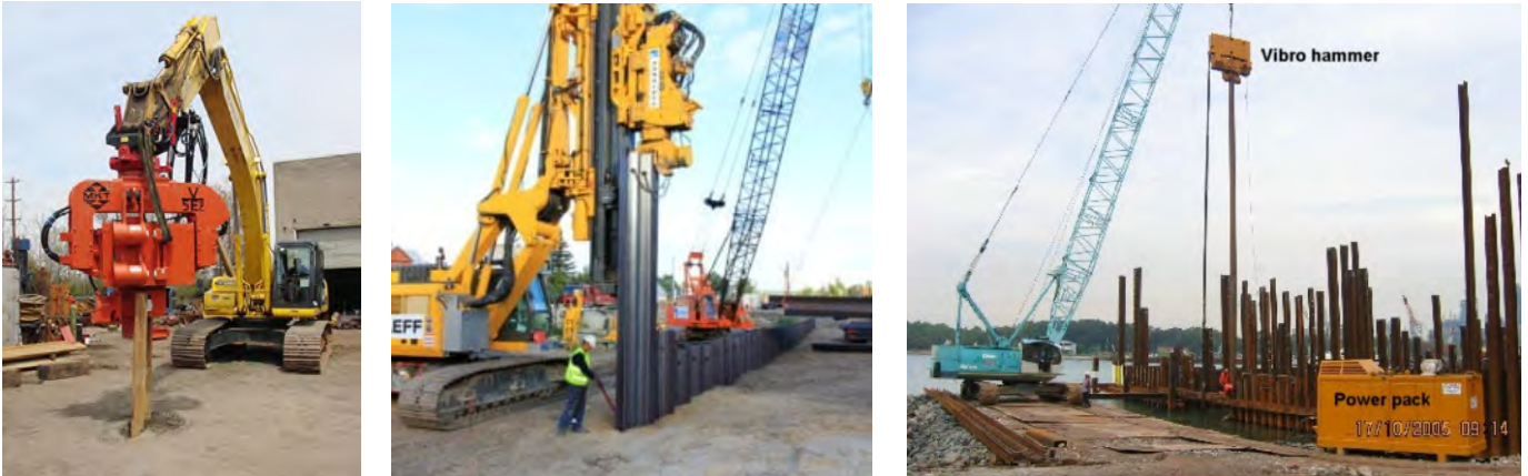
Figure 18.25: Typical Pile Installation Methods
