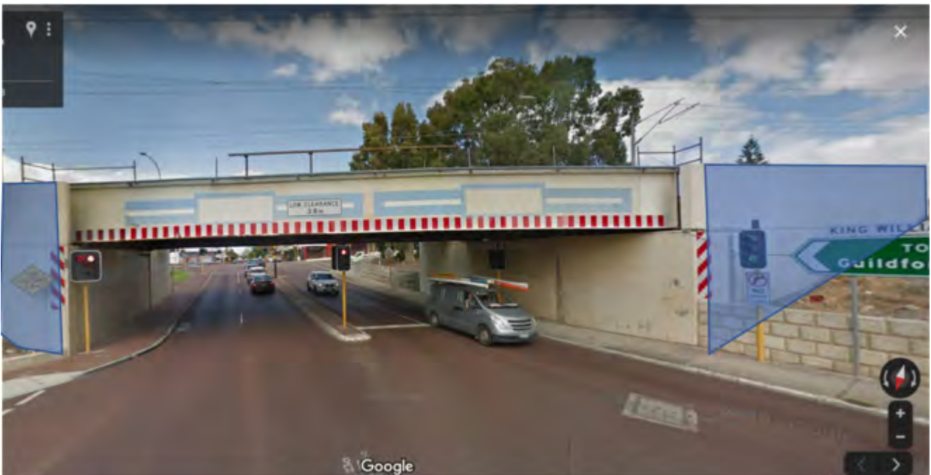
Figure 18.58: Wing Walls Demolition
