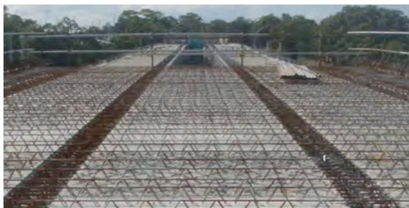
Figure 18.50: Transverse deck planks c/w structural “truss” reinforcement
