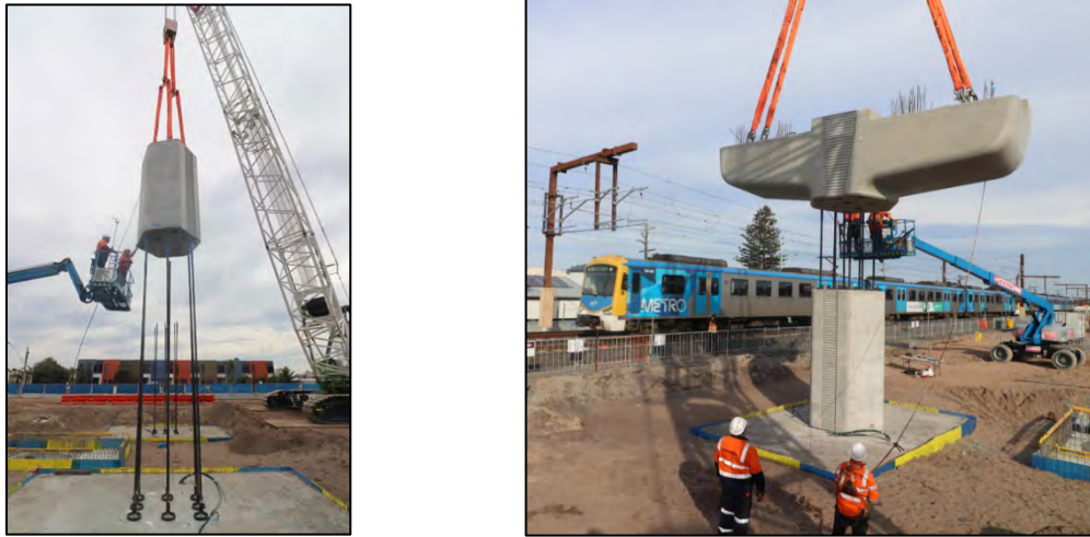
Figure 18.39: Pier Installation Photos
