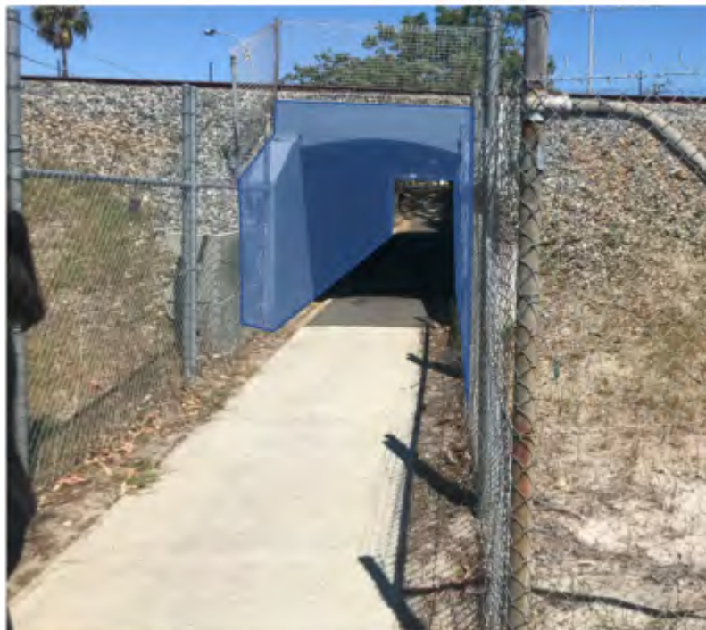
Figure 18.55: Leake Street Underpass Demolition
