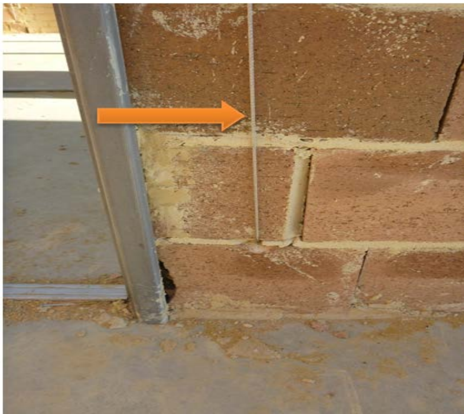
Figure 22. Photograph showing a hold-down wire attached into the internal masonry
