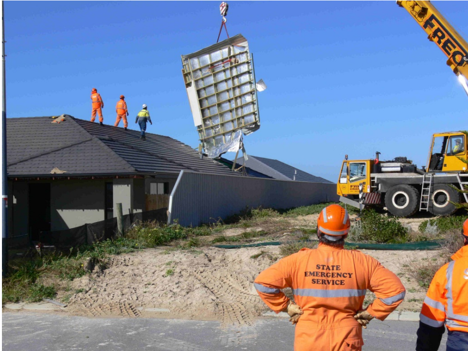
Figure 7. Photograph showing the result of a metal skillion roof lifting in high winds and landing on and damaging an adjoining property
