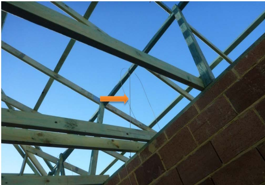
Figure 21. Photograph showing an internal hold-down wire fixed over underpurlin
