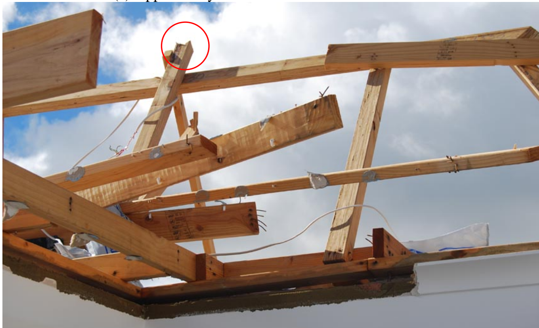
(b) Detail where parts of structure remained
