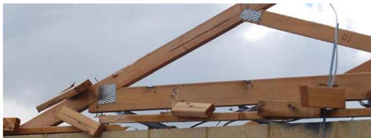
(b) lifting of timber top plate at truss heel joint
