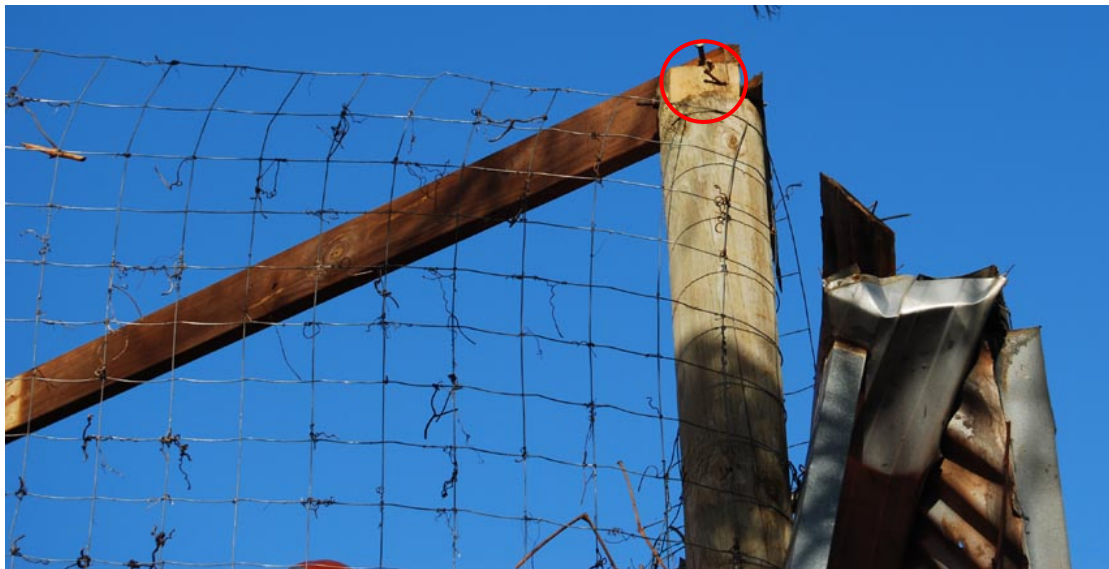
(b) Verandah post
