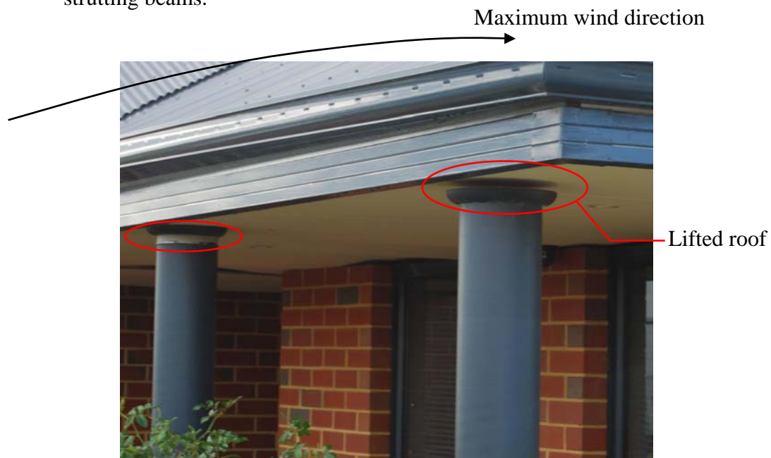
Figure 3.1 External (front) view of sheet roof house
