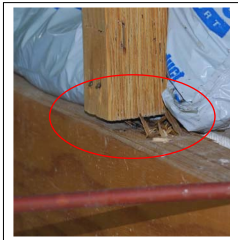
(b) connection at bottom of strut
