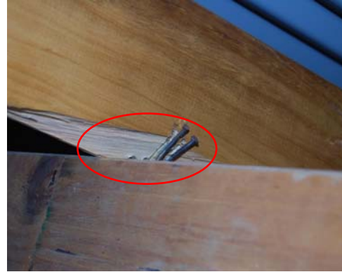
(b) rafter to top plate connection
