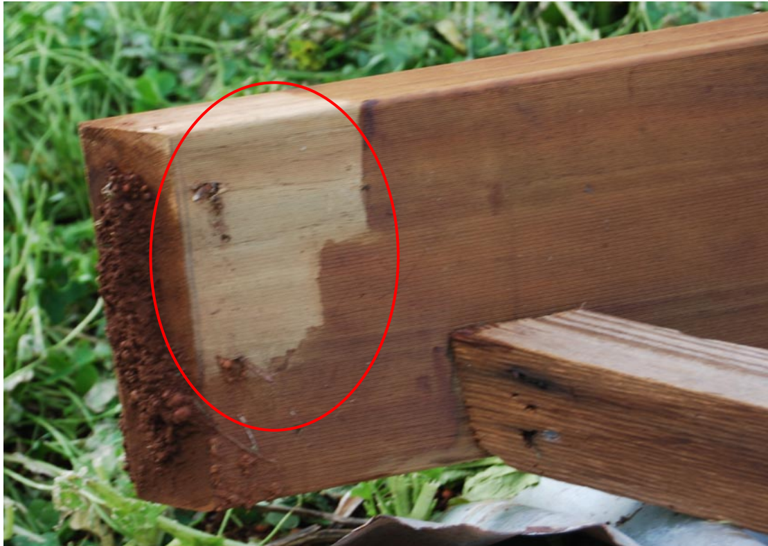
(a) Verandah beam
