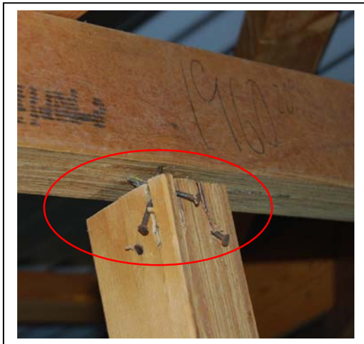
(a) connection at top of strut
