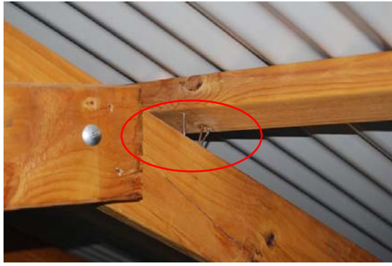
(a) batten to rafter connection
