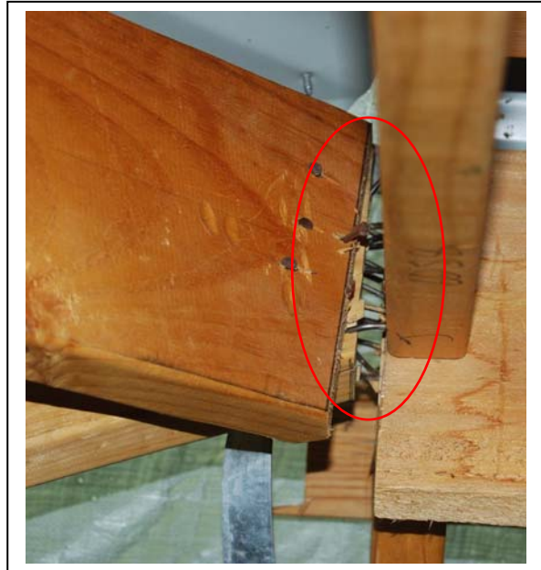
(c) connection at hip rafter
