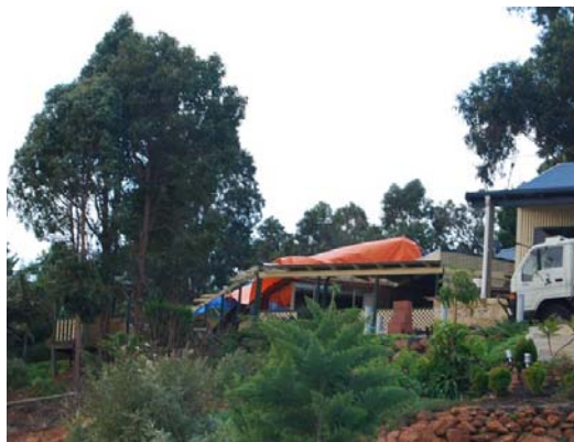
(a) Damage in first half of path
