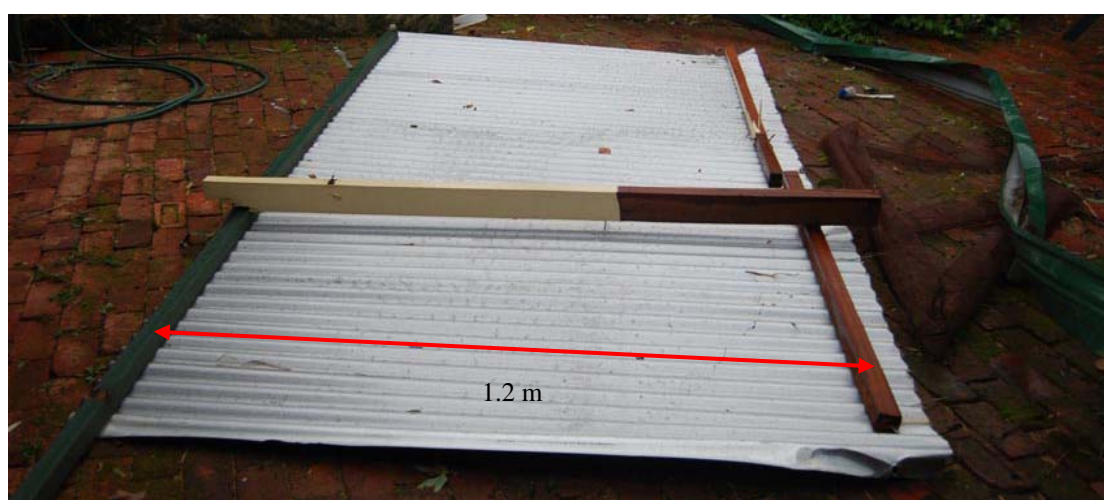
Figure 5.1 Batten spacing on verandah
