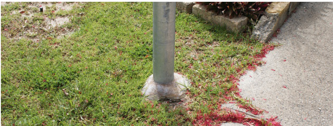
FIGURE 7 – CORRECT INSTALLATION OF STEEL POLE WITH CONCRETE FOOTING FINISHED ABOVE GROUND
