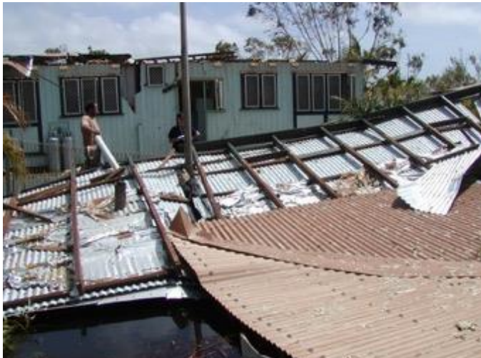
(c) Roofing and roof structure loss during a tropical cyclone in 2007. The original metal sheet roof had been tied-down with over-battens, which were removed, and the tie-down rods were cut when the roof was replaced. No alternative tie-down system was installed.
