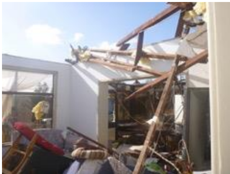
(d) Damage to a two-storey house built in 1964. The original tile roof was replaced with a metal sheet roof in 2002. The roof cladding and roof structure were lost during a storm in 2014.
