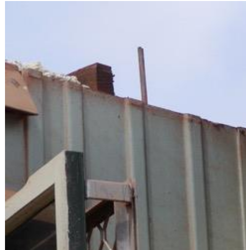
(c) Roofing and roof structure loss during a tropical cyclone in 2007. The original metal sheet roof had been tied-down with over-battens, which were removed, and the tie-down rods were cut when the roof was replaced. No alternative tie-down system was installed.
