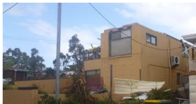
(d) Damage to a two-storey house built in 1964. The original tile roof was replaced with a metal sheet roof in 2002. The roof cladding and roof structure were lost during a storm in 2014.
