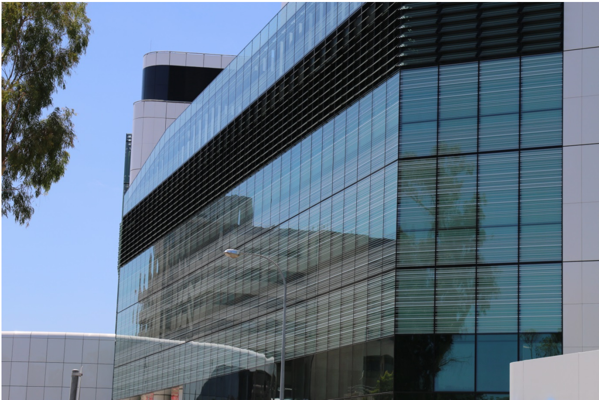
Photograph 14: Curtain wall glazing at Perth Children's Hospital
