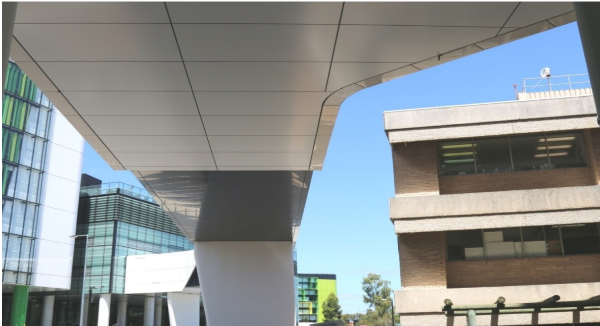
Photograph 10: Alucobond Plus panels under the link bridge
