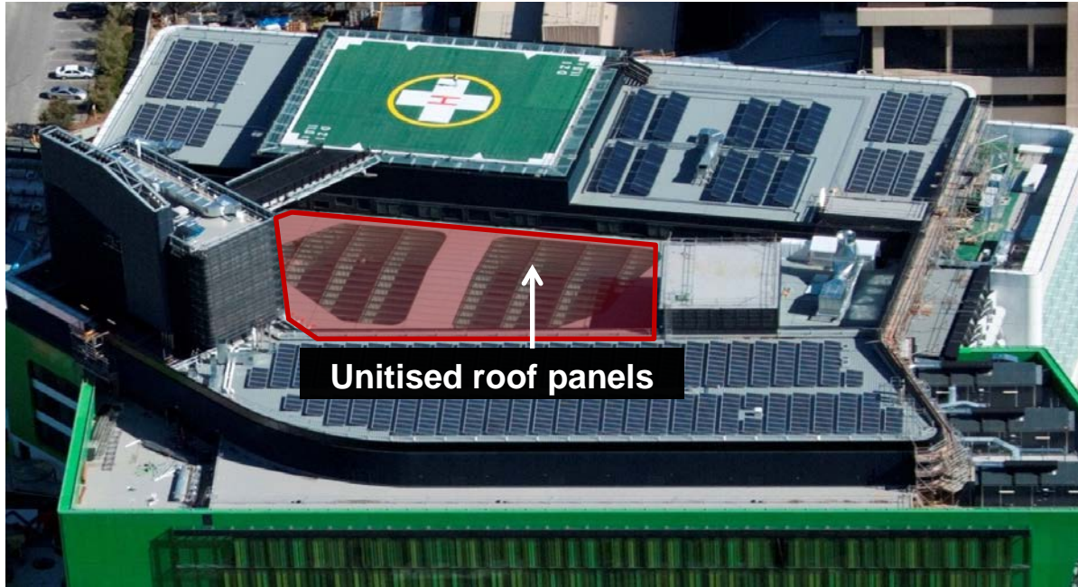
Photograph 2: Helipad and unitised roof panels at Perth Children’s Hospital
