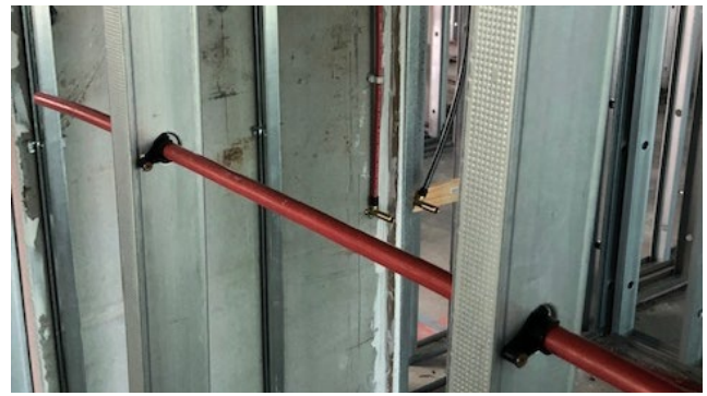
Photo 6: Compliant clipping in metal framework.
